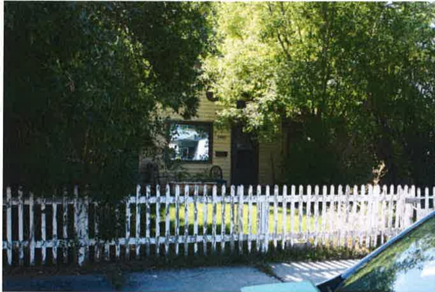
Subject: 1020 Terry Ave., Billings, MT 59102 Description: Front façade; photographer facing south
