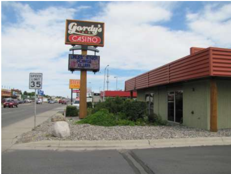
View east down Grand Ave
