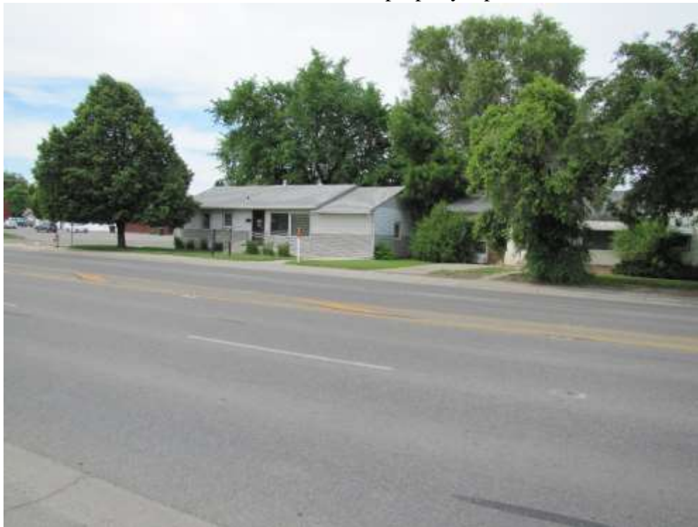
View north and west across Grand Ave
