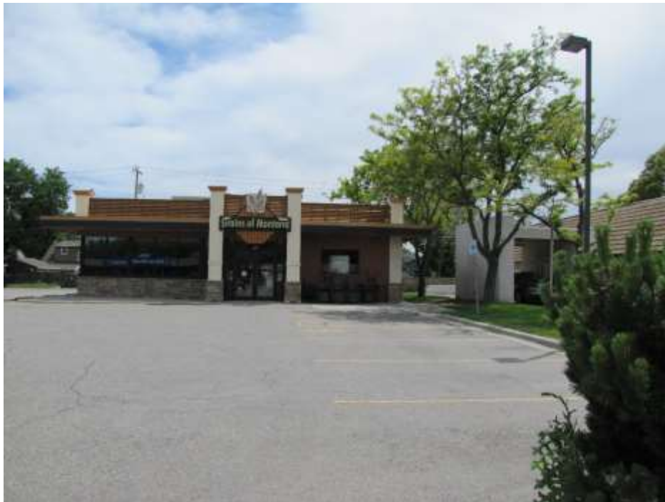
Front façade at 926 Grand – subject property
