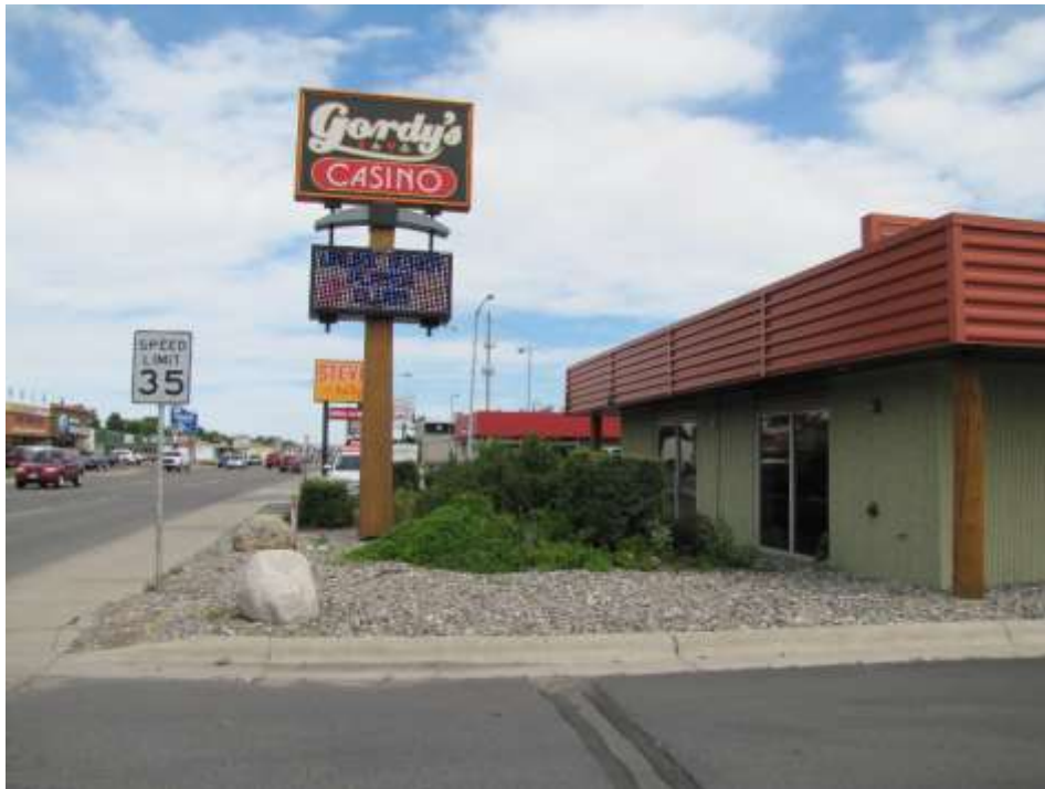
View east down Grand Ave
