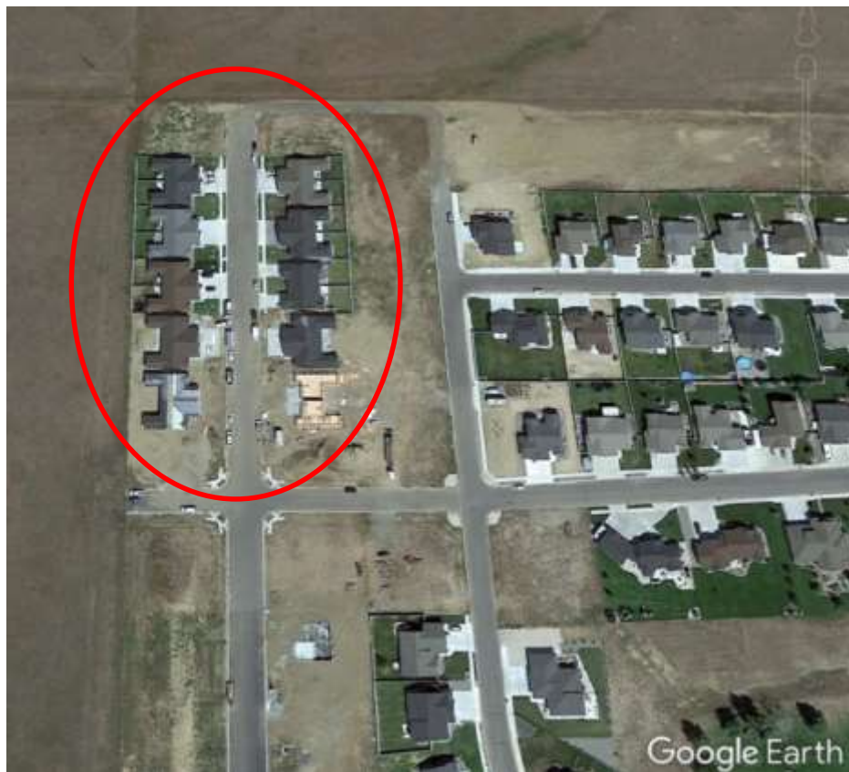
Builder's current townhome project on the north end of Gleneagles Blvd
