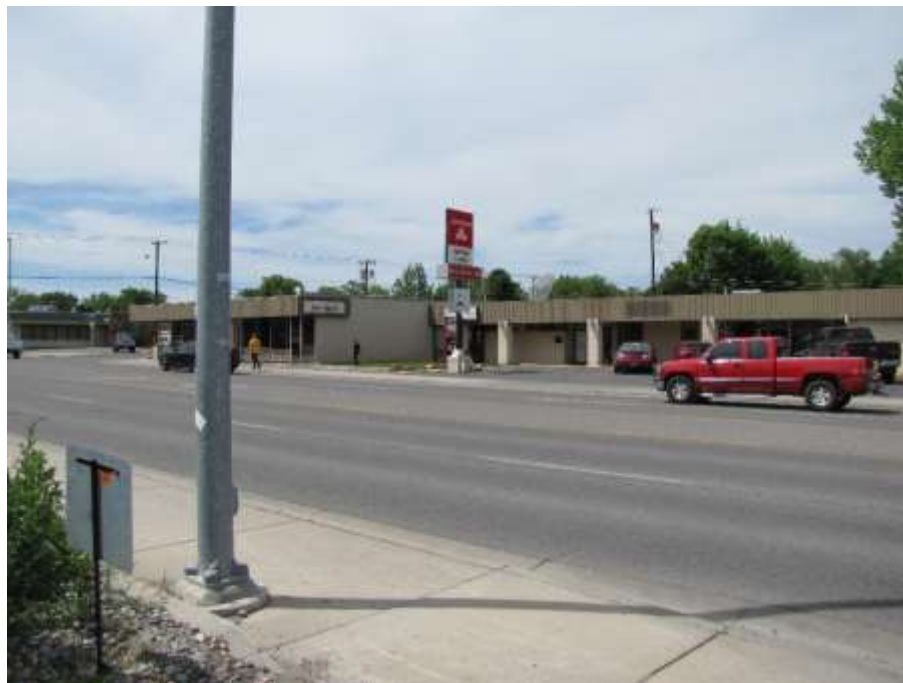
View north and west across Grand Ave
