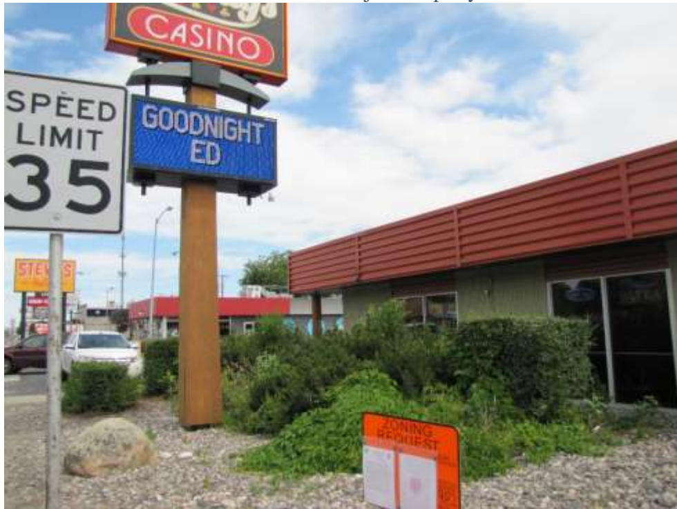
Front façade at 2244 Grand – subject property
