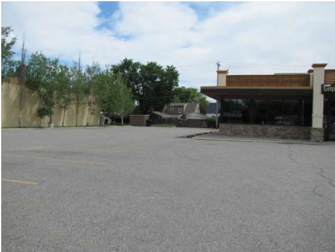
View south across subject property to open alley access
