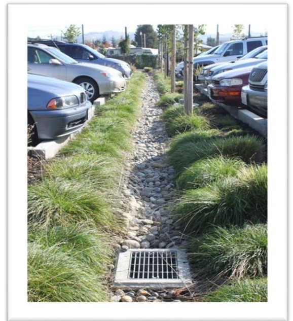
Fig. 27-1200.F Left: Landscape islands with storm water infiltration.
