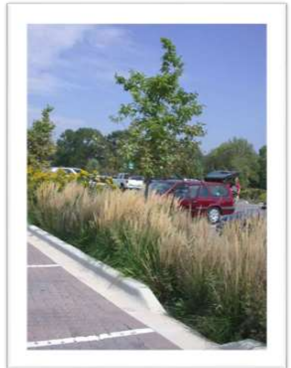
Fig. 27-1200.G: Curb cut to allow drainage
