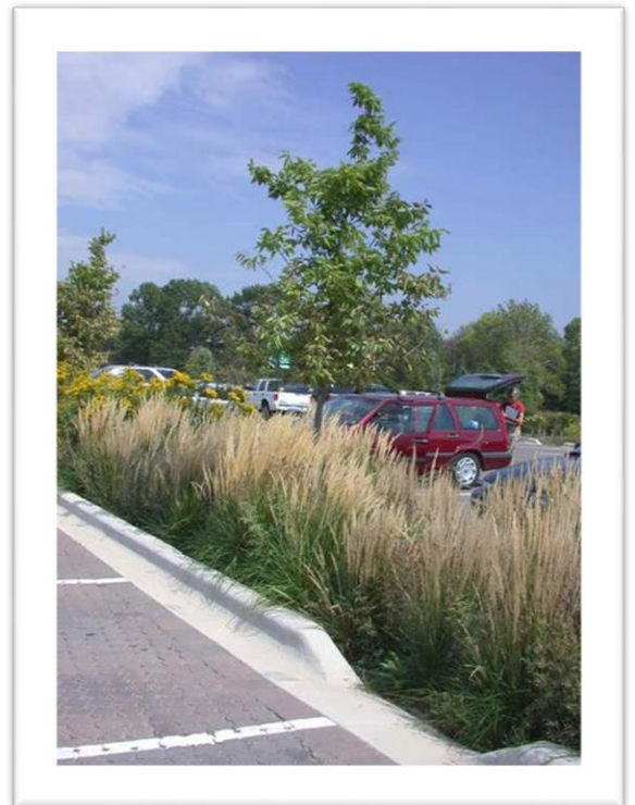
Fig. 27-1200.H: Curb cut to allow drainage
