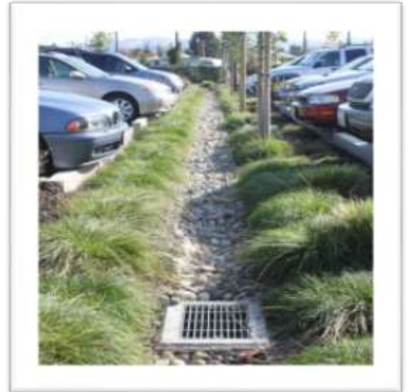
Fig. 27-1106.B Left: Landscape islands with storm water infiltration;
