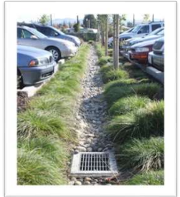
Fig. 27-1200.E Left: Landscape islands with storm water infiltration.
