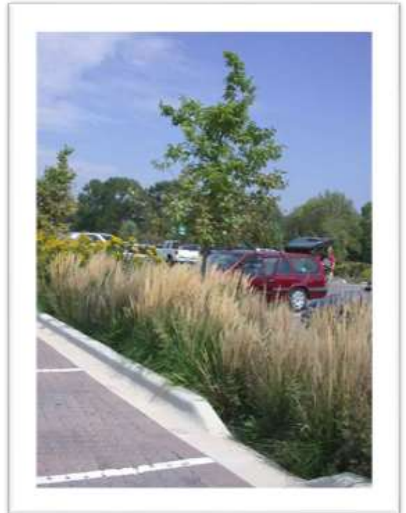
Fig. 27-1200.G: Curb cut to allow drainage
