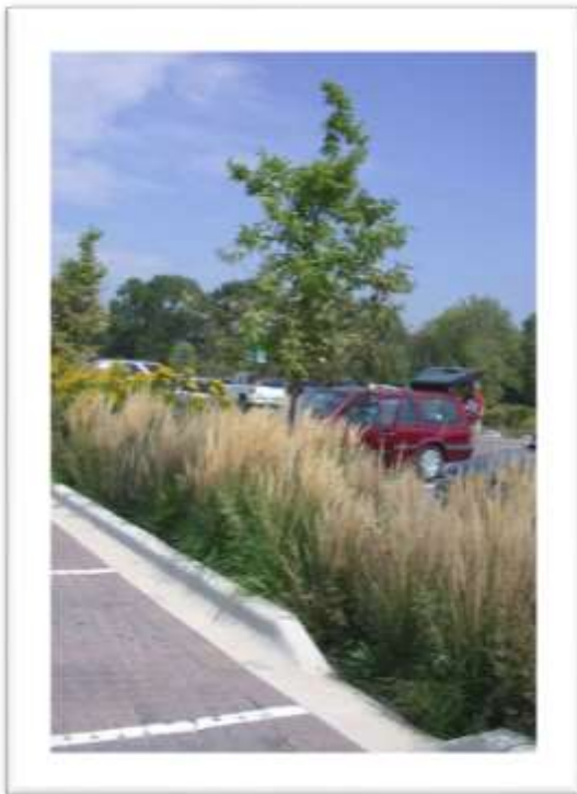
Fig. 27-1106.D: Curb cut to allow drainage
