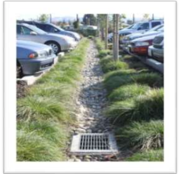
Fig. 27-1106.B Left: Landscape islands with storm water infiltration;
