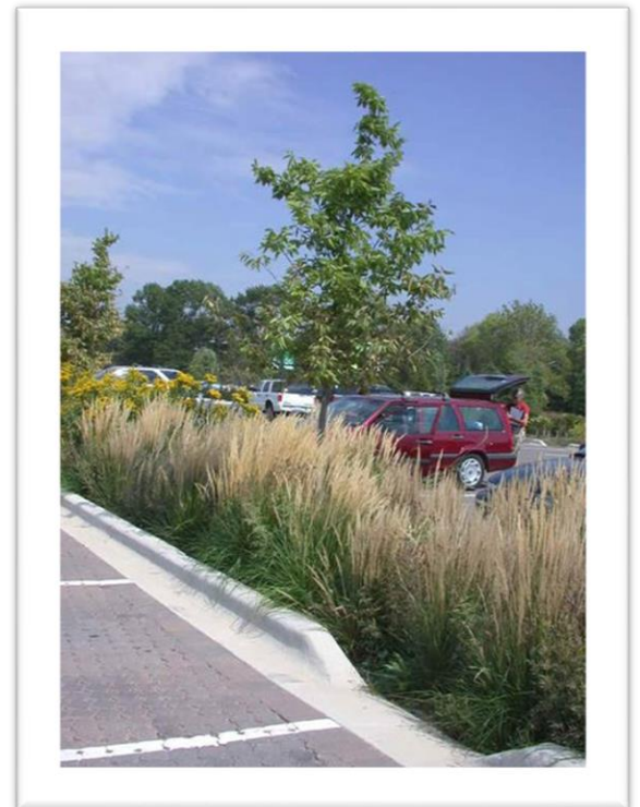
Fig. 27-1200.H: Curb cut to allow drainage
