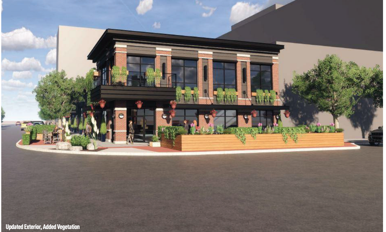
Main Floor Patio, Second Floor Balcony and Rooftop Patio
