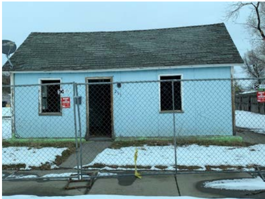
213 North 20 th Street Front View – Looking East
