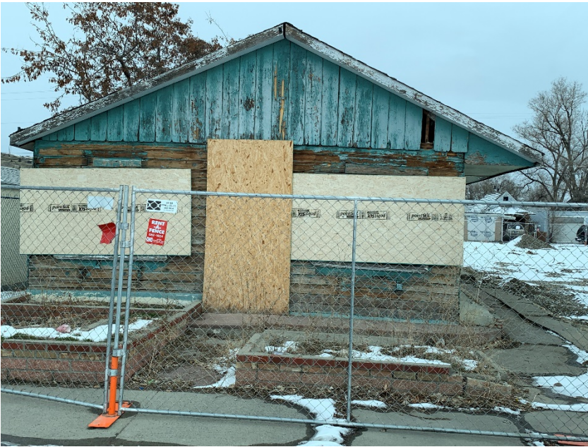
219 North 20 th Street Front View – Looking East
