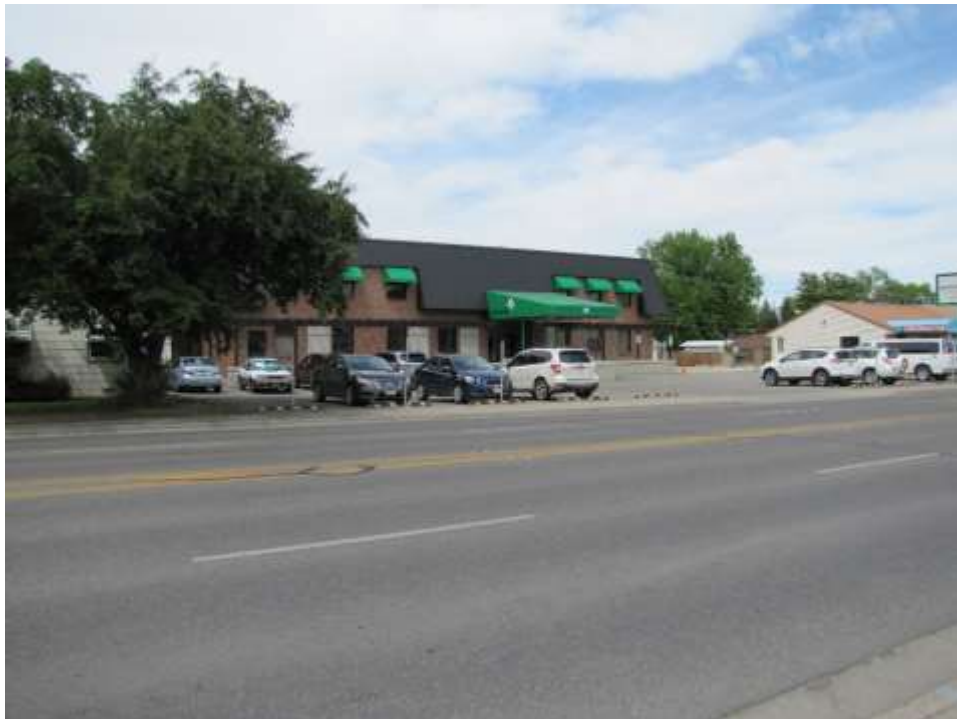
View north and east across Grand Ave
