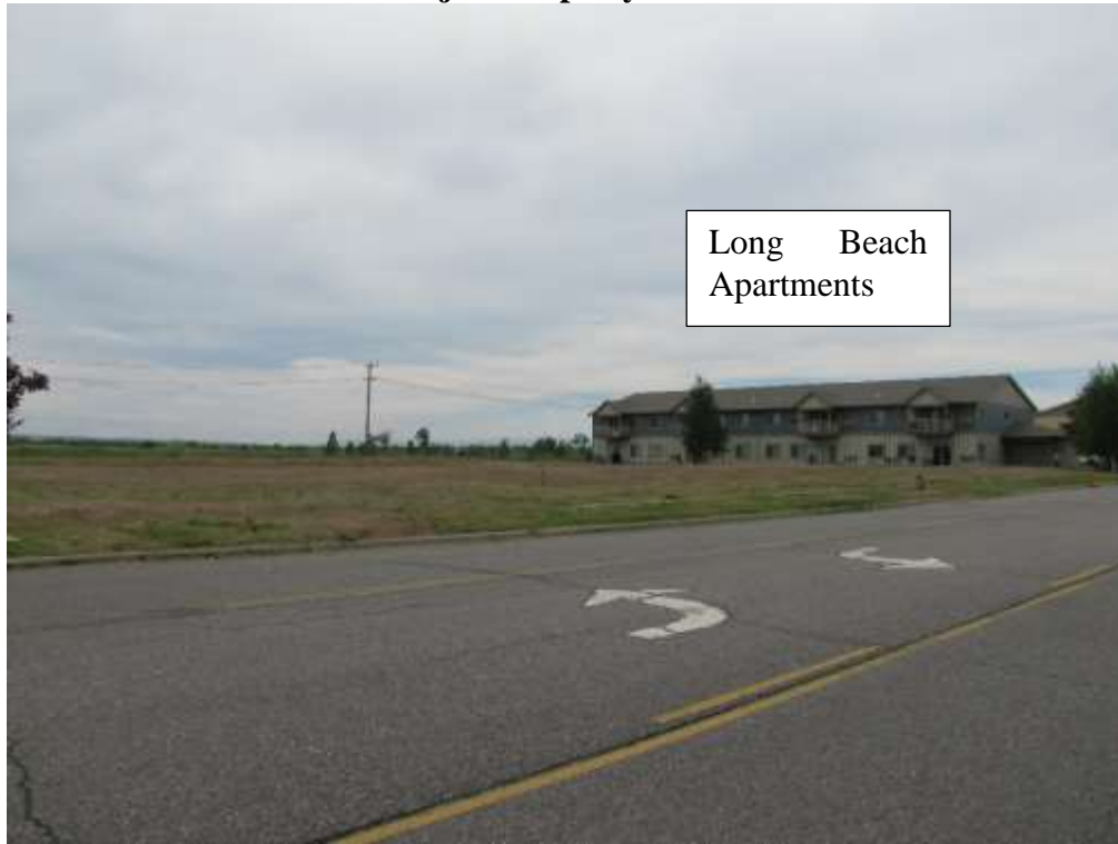
View south and west across Montana Sapphire Dr
