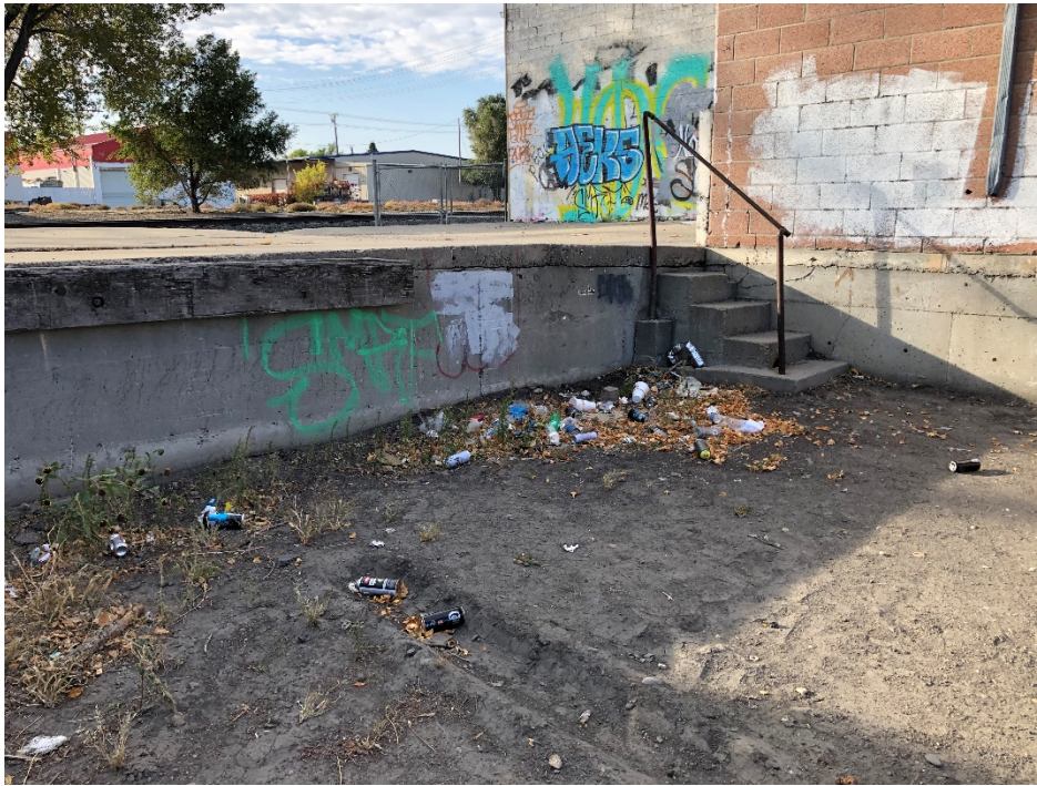
Loading dock at Subject Property at 501 North 22 nd Street.
