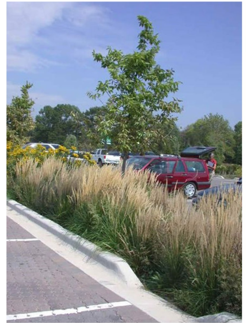
Fig. 27-1200.G: Curb cut to allow drainage
