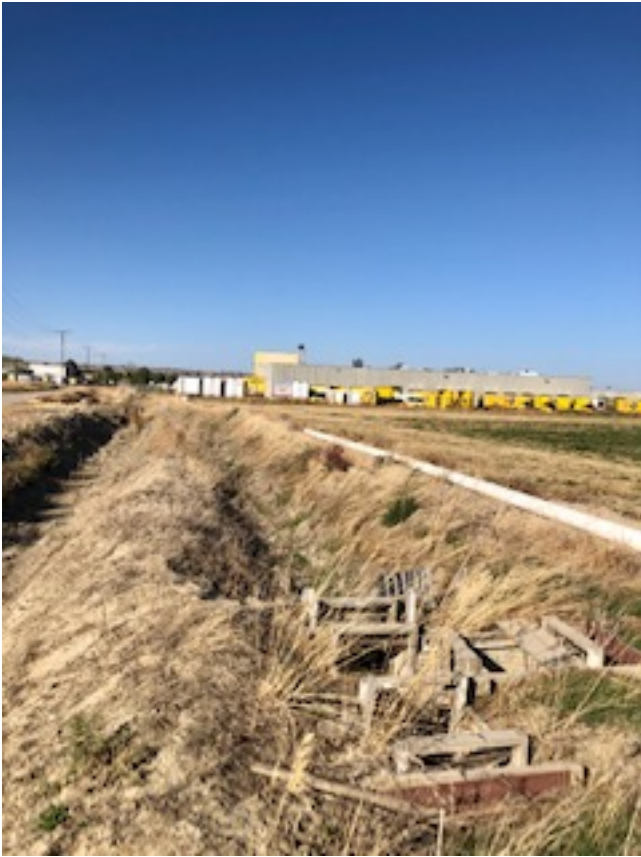
View from southwest corner of site looking north
