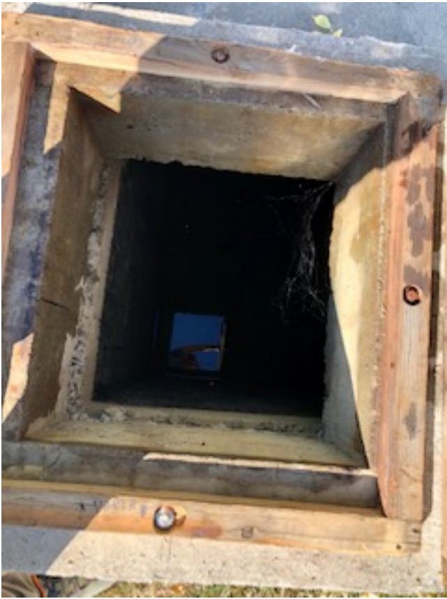
View looking down into GW well cistern – backyard
