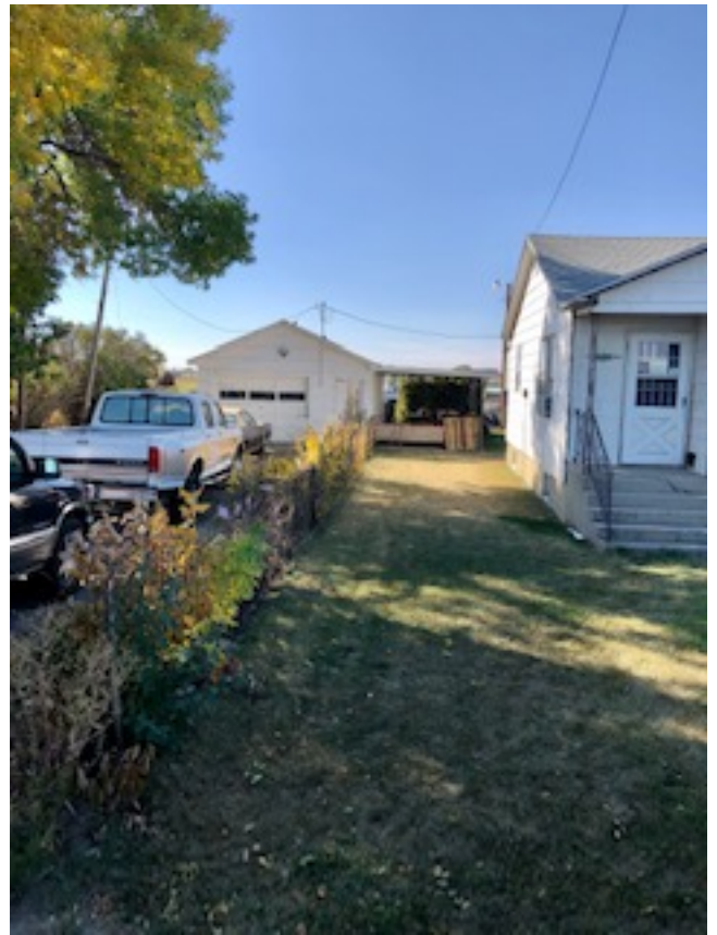
View from west looking site home and garage
