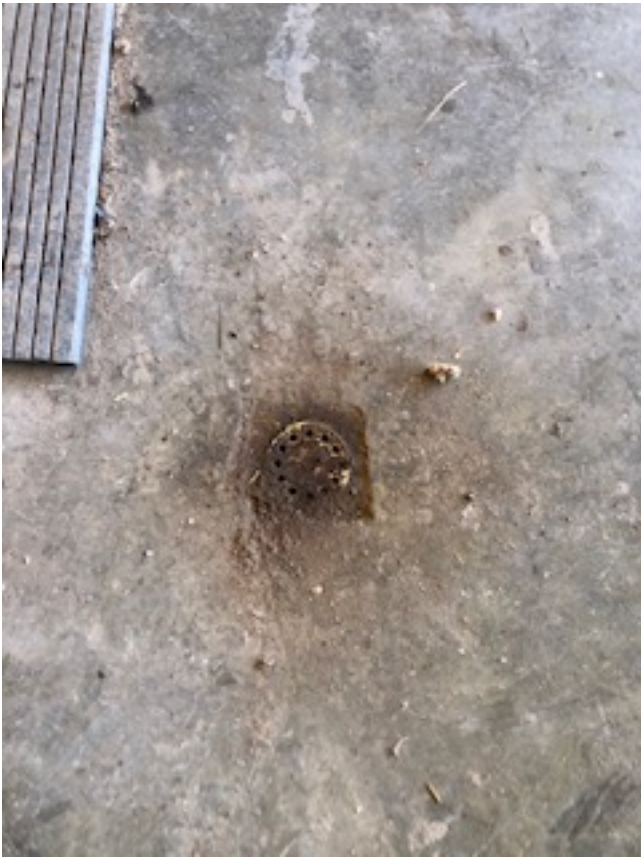
View of shop floor drain 2 – close-up
