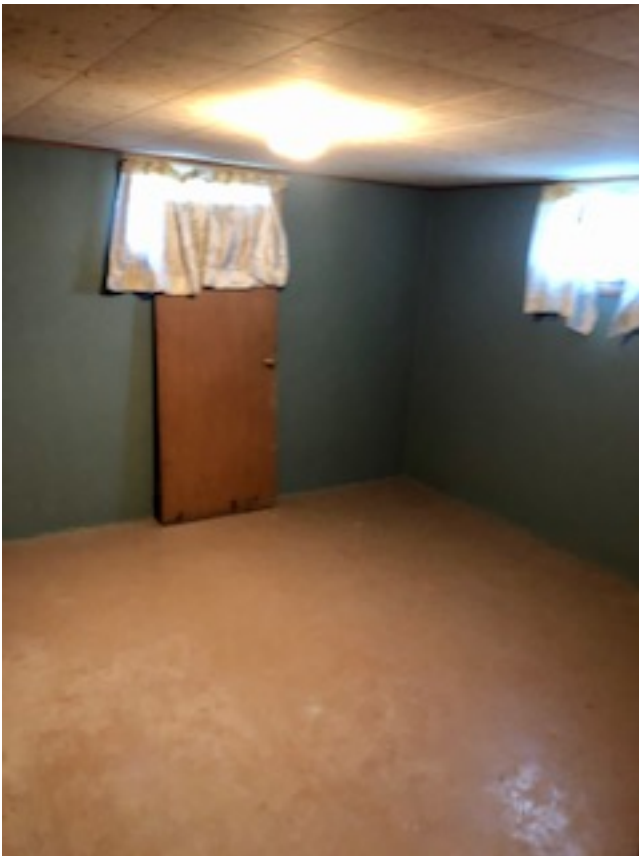
View of bedroom 4 – northeast corner of basement
