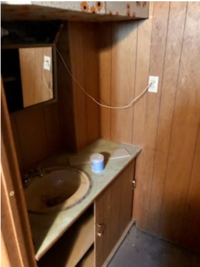
View of bedroom 4 closet area with sink.
