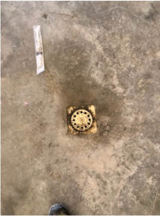
View of shop floor drain 1 – close-up
