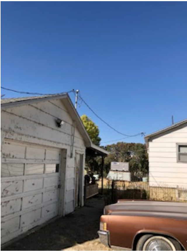
View on west side of garge looking north
