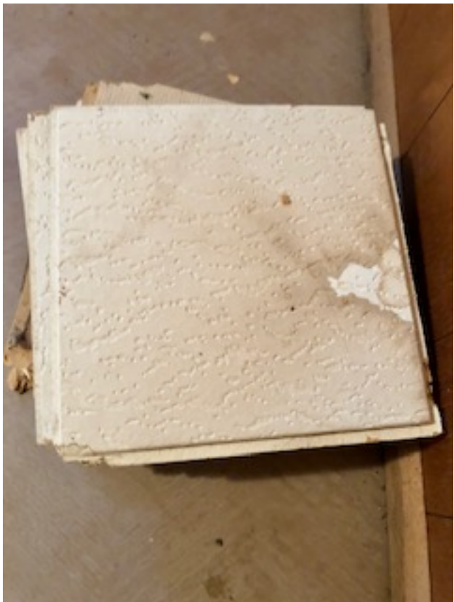
Old, false ceiling tiles located in basement – NE bedroom
