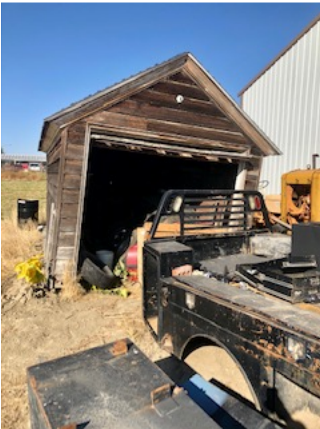
View of shed on west side of shop
