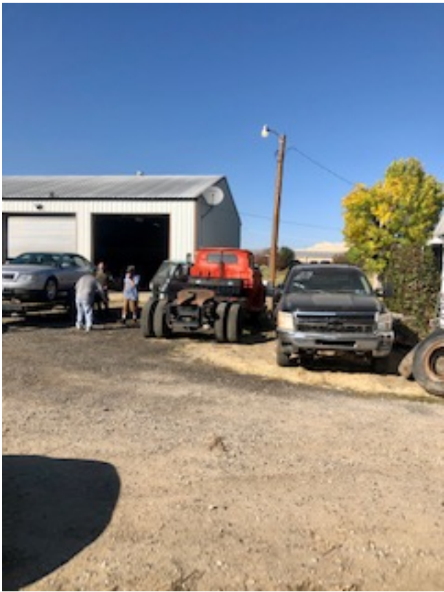
View looking north at the site shop building
