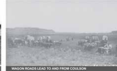
WAGON ROADS LEAD TO AND FROM COULSON
