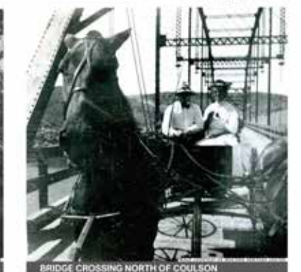
BRIDGE CROSSING NORTH OF COULSON
