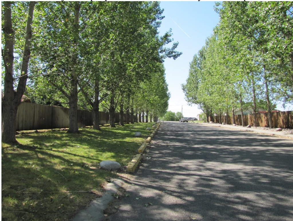
View west to intersection of Cherry Creek Loop & Bitterroot Drive
