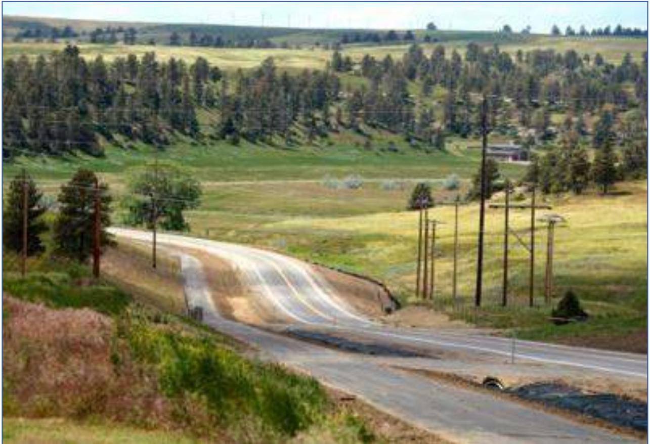
Skyway Drive (Phase 1 of the Inner Belt Loop) opened to traffic in 2014
