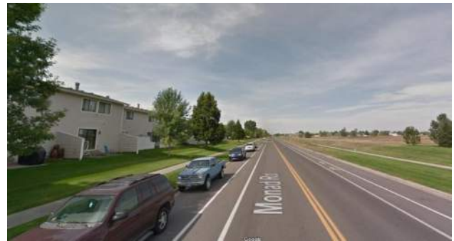
Option 1: Development along Monad Road in Billings shows a shallow setback with apartments close to the right-of-way
