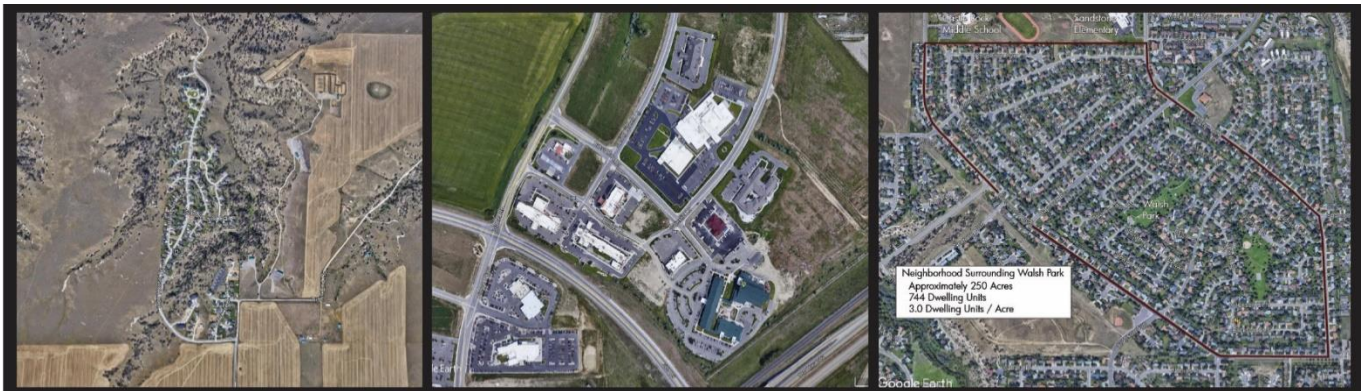
Aerial images showing examples placed used to generate density and FAR assumptions. Rehberg Ranch, Gabel Road, and a Billings Heights neighborhood
