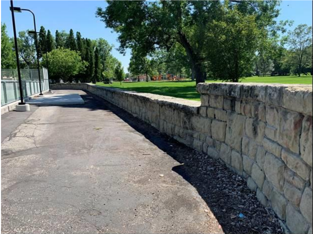
MT_YellowstoneCounty_PioneerPark_0018 View of northern tennis courts retaining wall, view looking southwest
