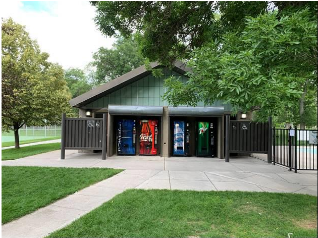
MT_YellowstoneCounty_PioneerPark_0028 View of restrooms, view looking west
