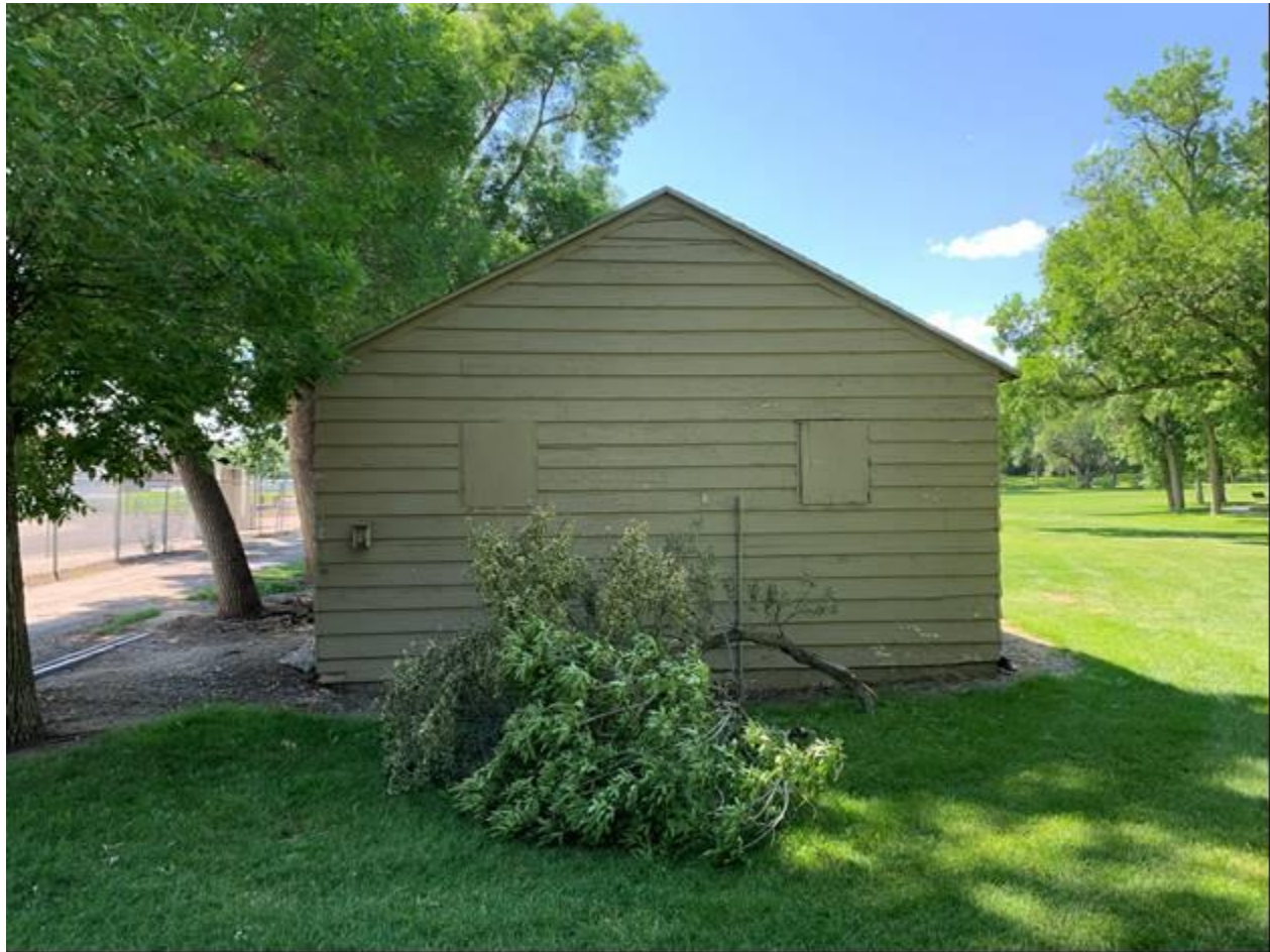
MT_YellowstoneCounty_PioneerPark_0040 View of park storage facility, view looking west
