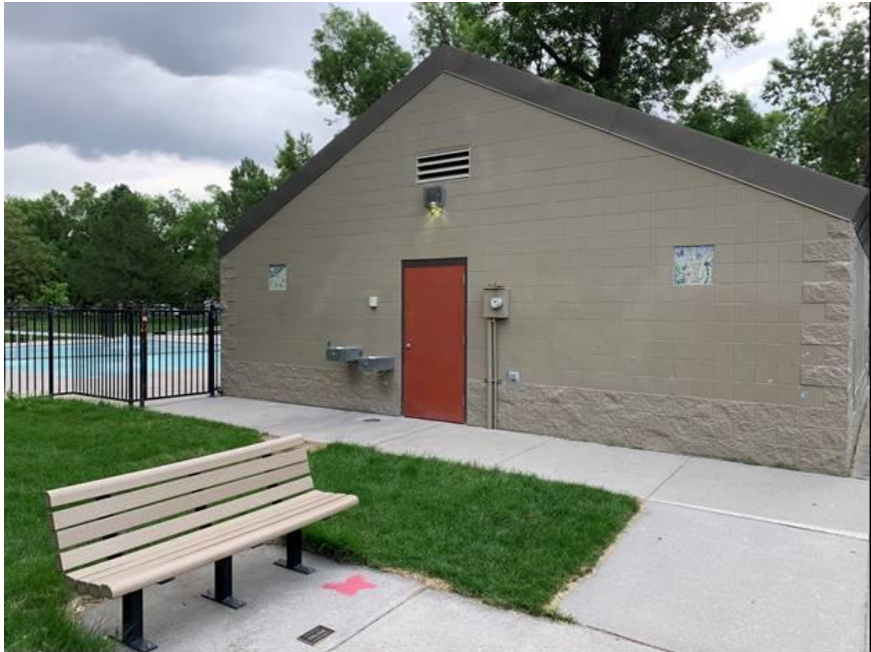
MT_YellowstoneCounty_PioneerPark_0029 View of restrooms, view looking northeast
