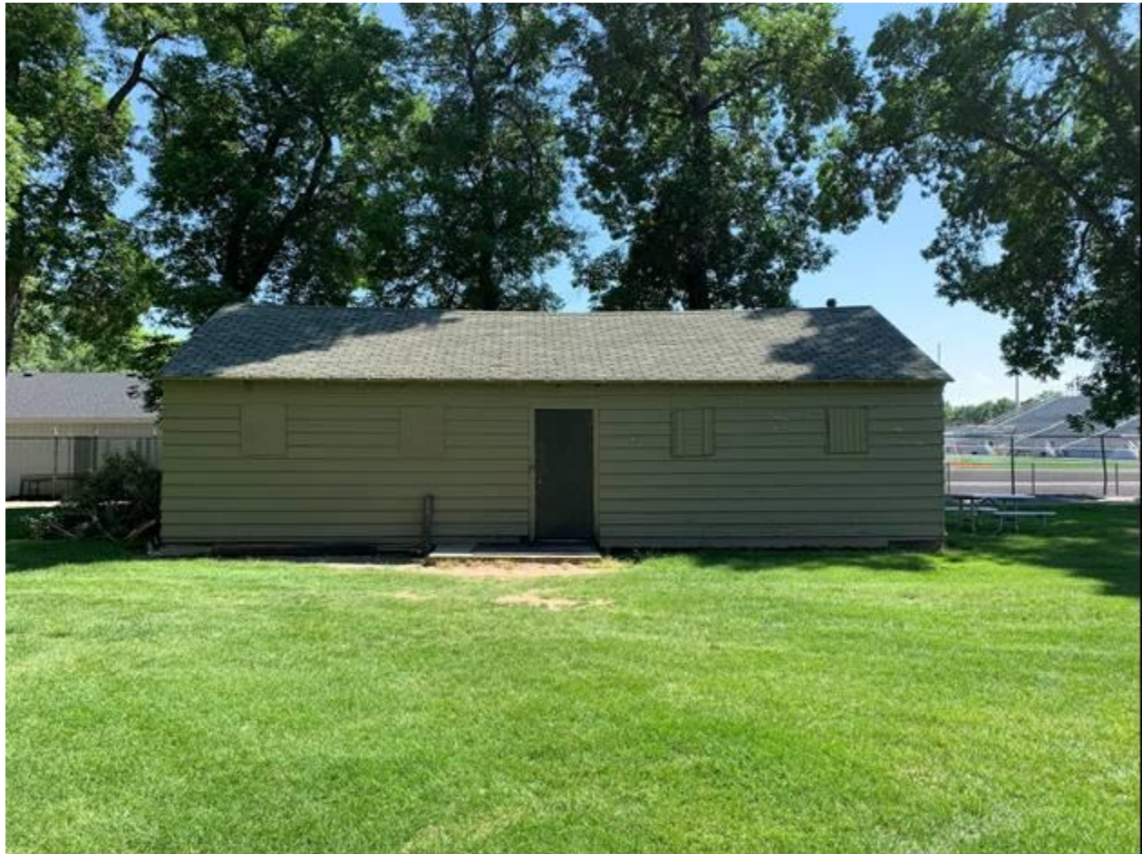
MT_YellowstoneCounty_PioneerPark_0037 View of park storage facility, view looking south
