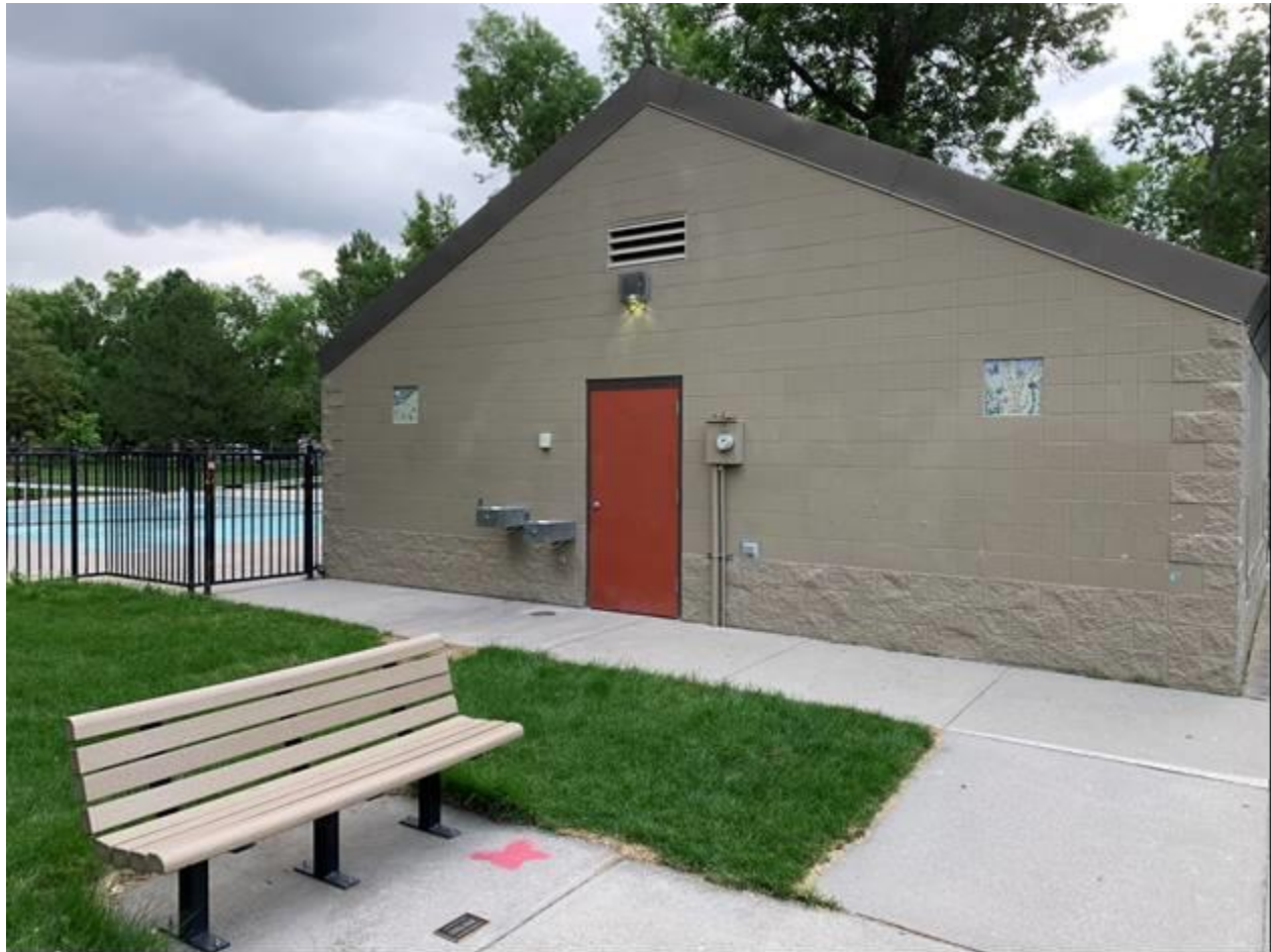
MT_YellowstoneCounty_PioneerPark_0029 View of restrooms, view looking northeast
