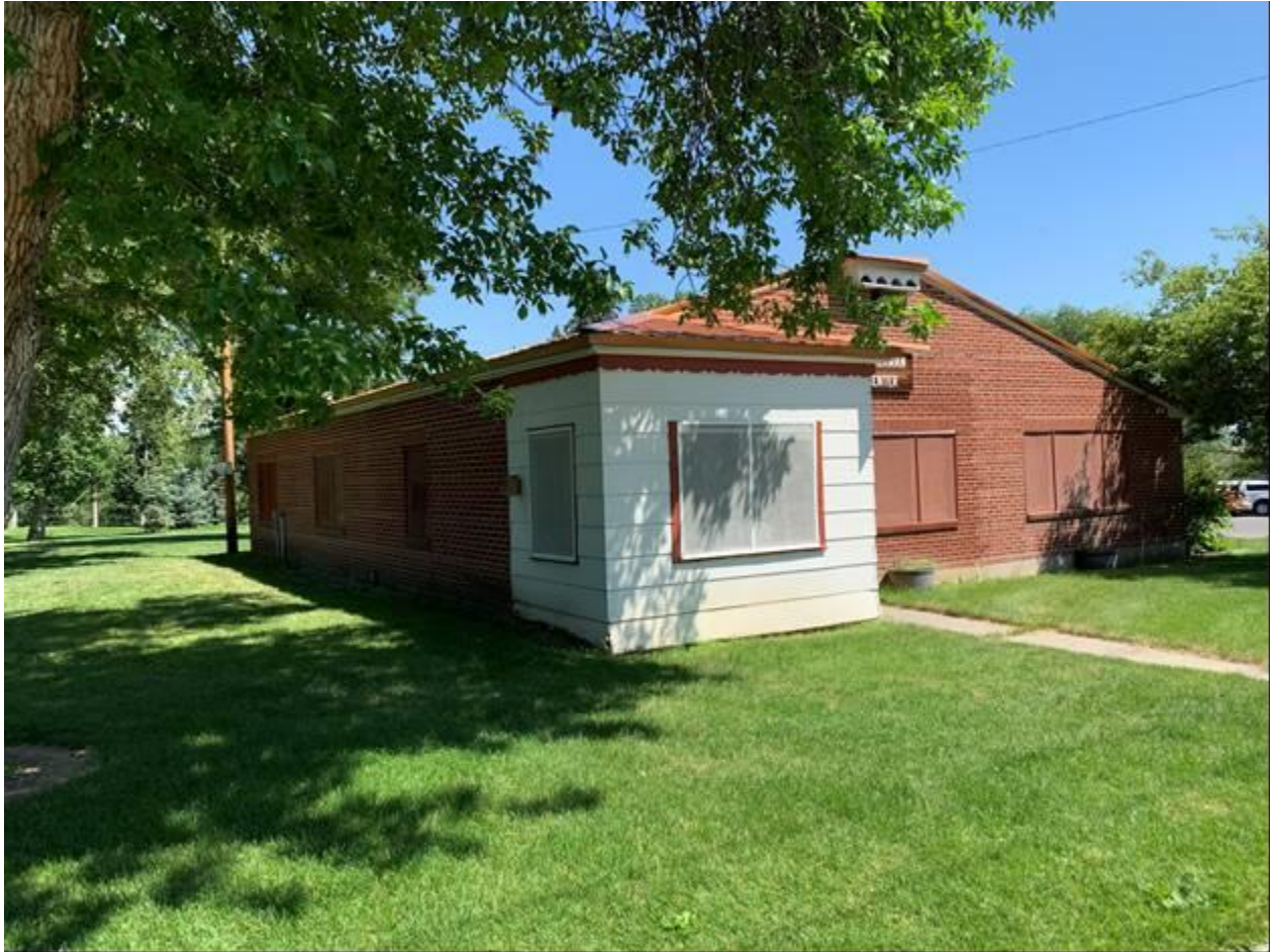
MT_YellowstoneCounty_PioneerPark_0003 Zimmerman Center, view looking southeast
