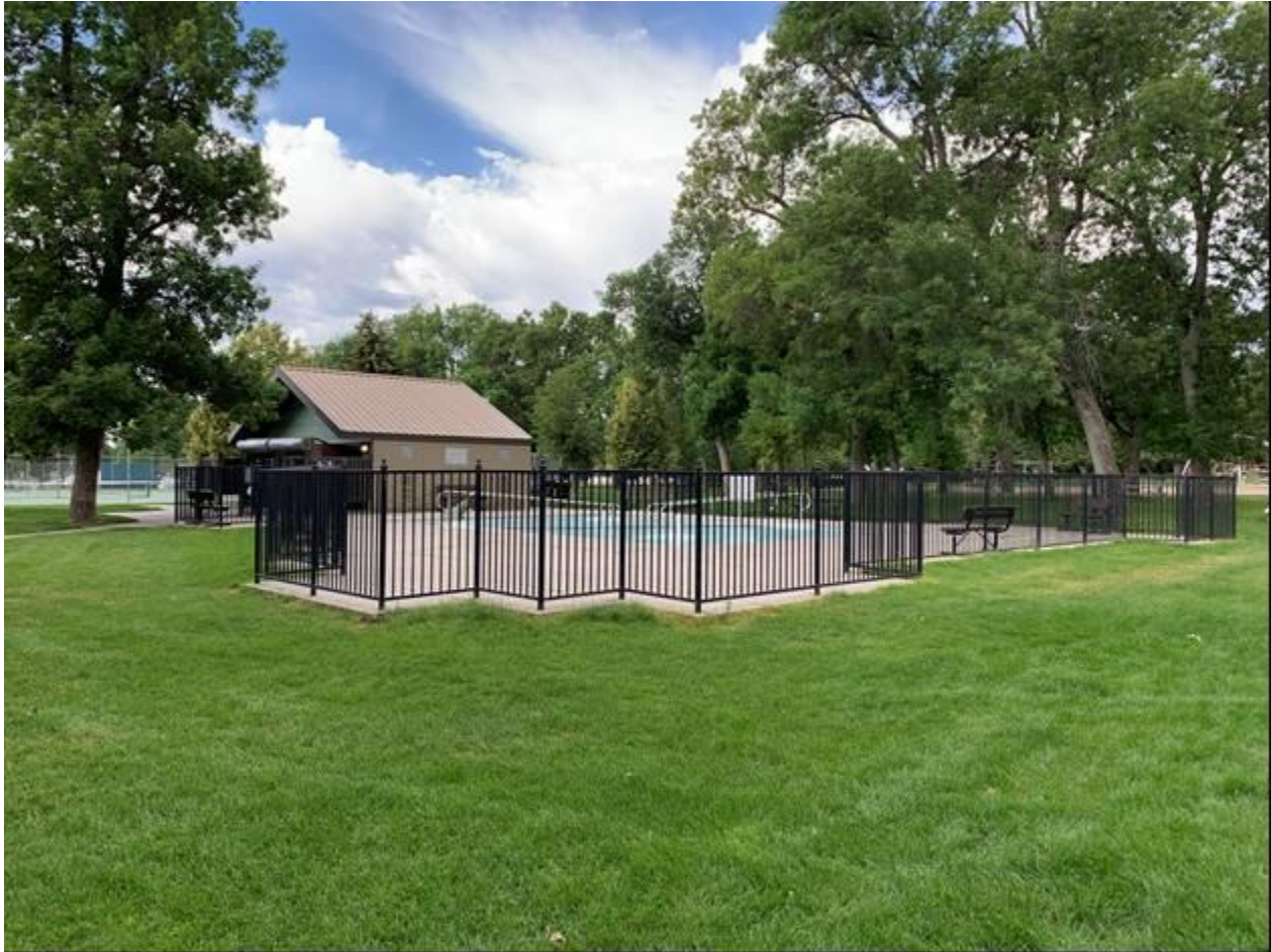
MT_YellowstoneCounty_PioneerPark_0026 View of wading pool area, view looking southwest
