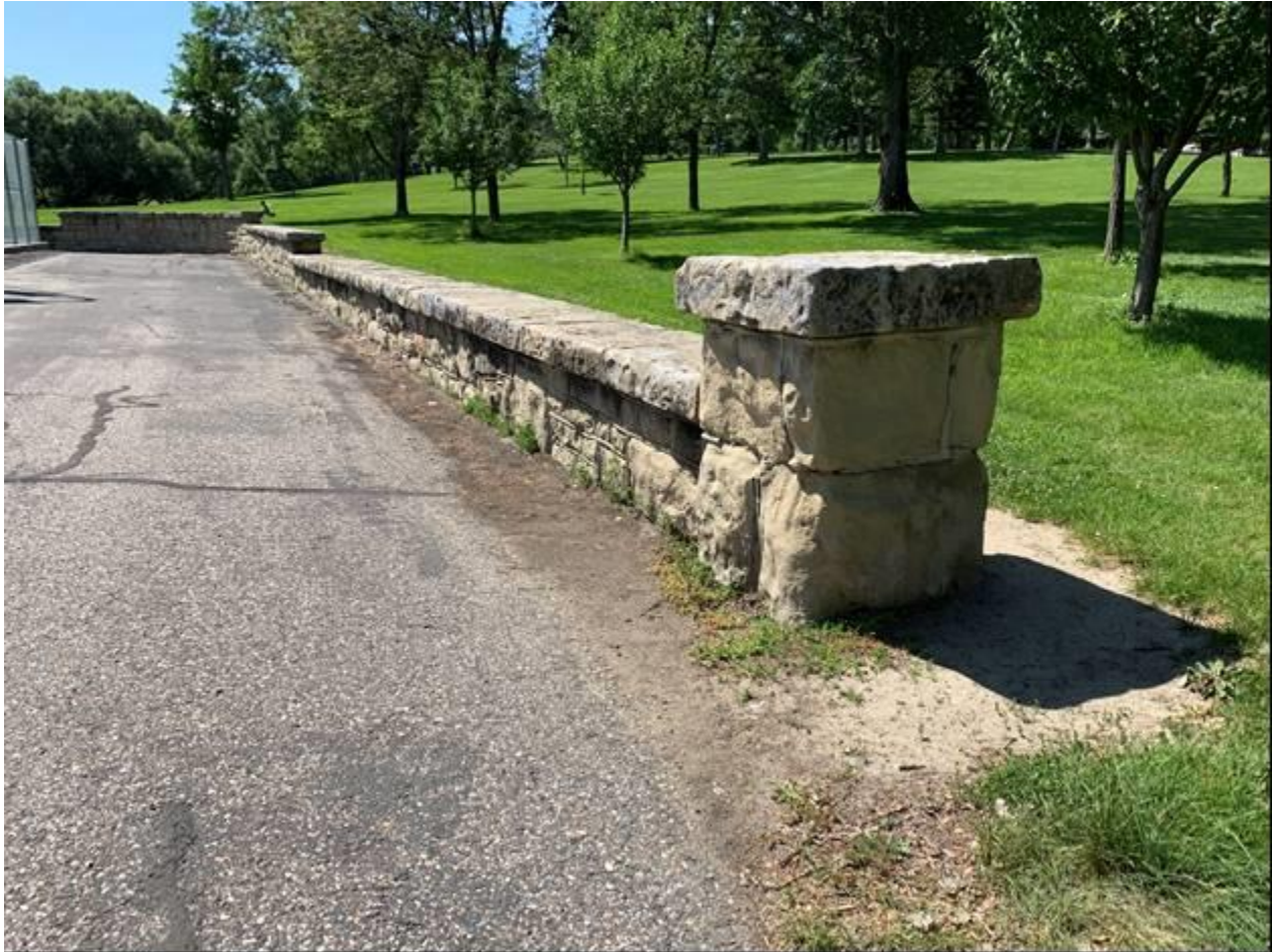
MT_YellowstoneCounty_PioneerPark_0016 View of northern tennis courts retaining wall, view looking west
