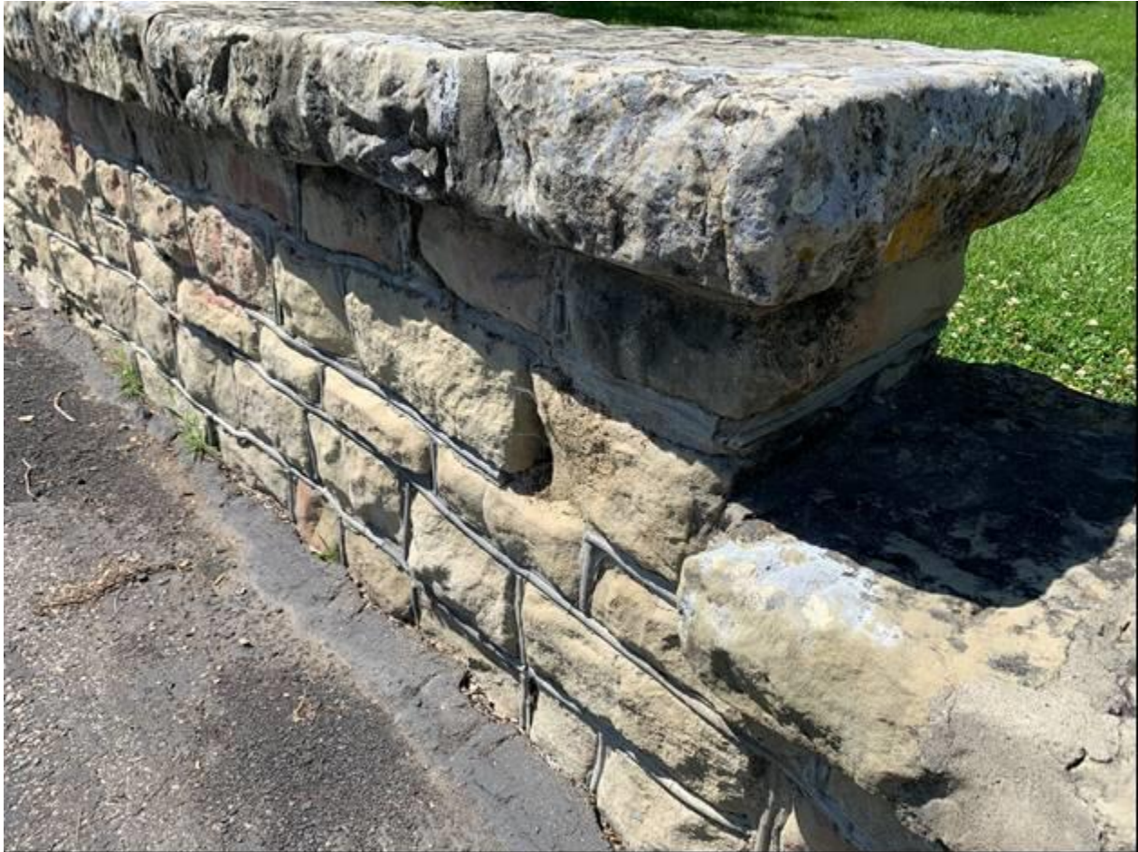
MT_YellowstoneCounty_PioneerPark_0017 View of northern tennis courts retaining wall, view looking northwest
