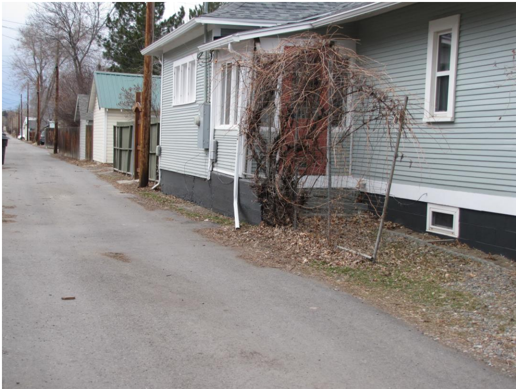
Looking West on the South side of the house
