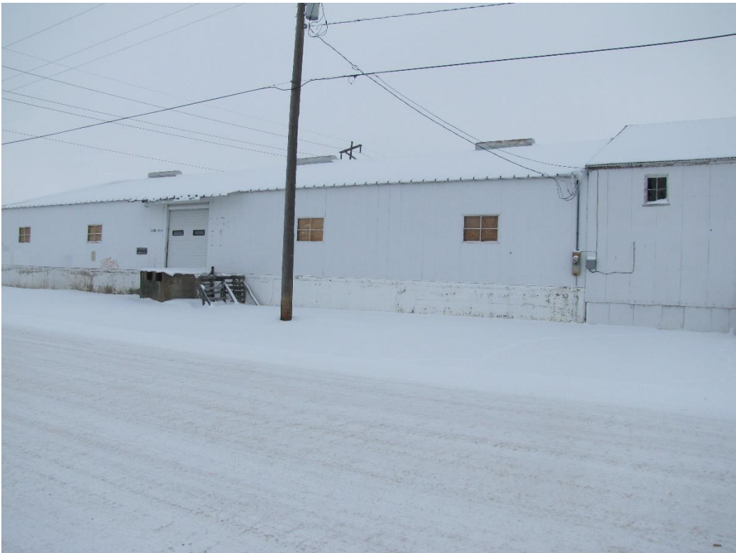
View south across Montana Avenue
