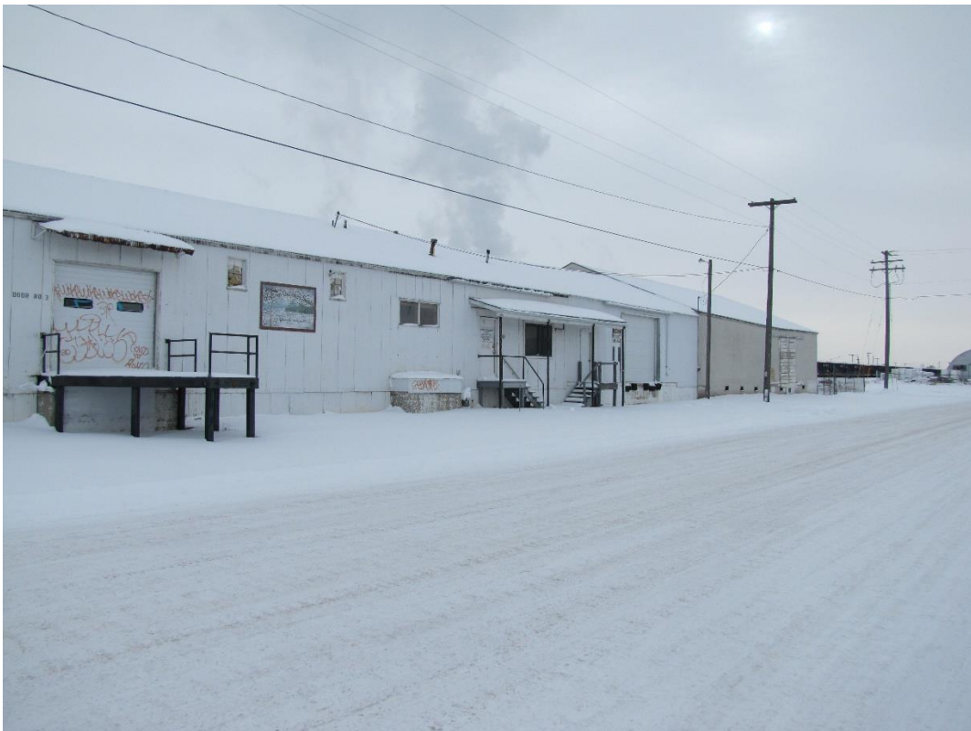
View south and west across Montana Avenue
