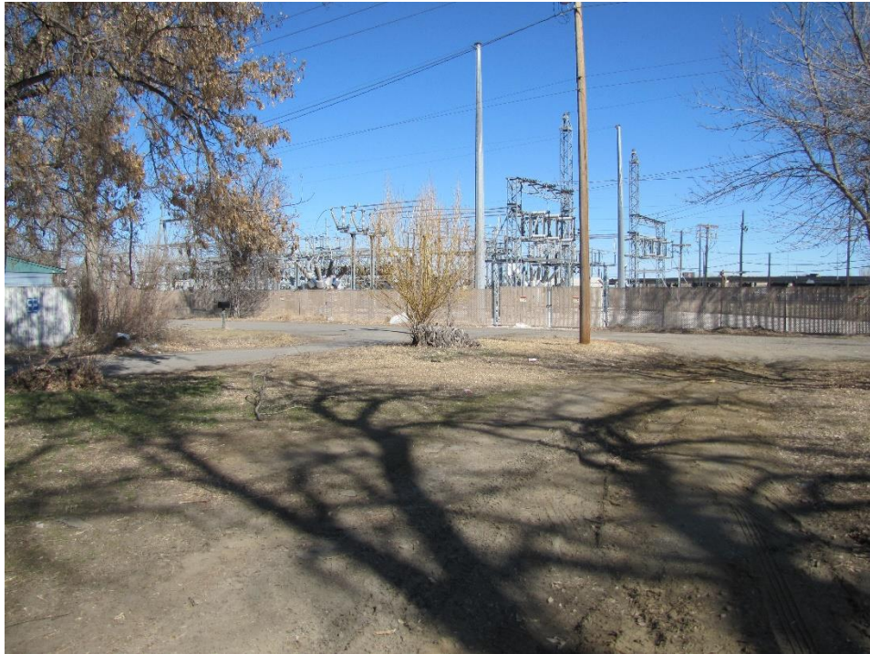
View north and west from dead end of Rhea Lane
