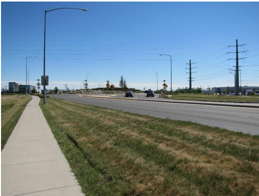
View of roundabout at King Ave W and Shiloh Road
