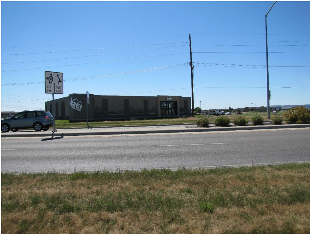
View west across Shiloh Road at REI in St Vincent's Healthcare Subdivision
