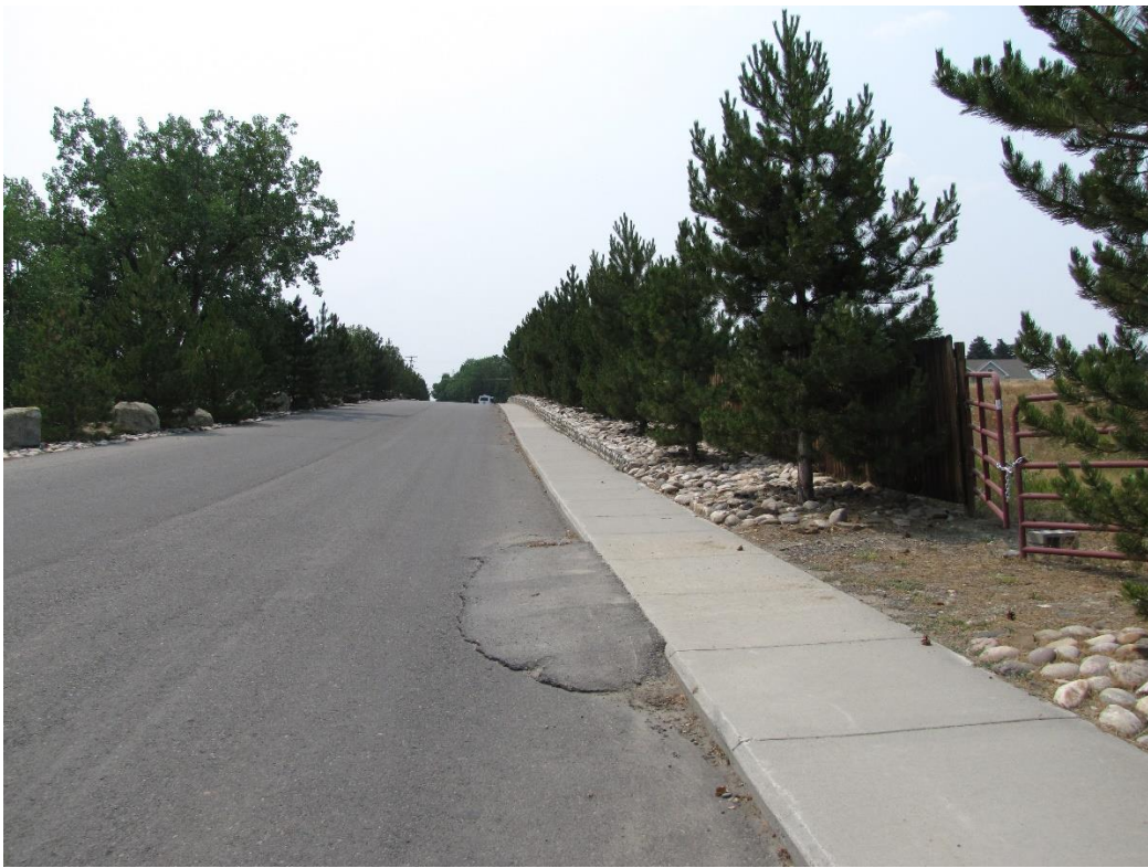
View west along southern leg of Cherry Creek Loop – subject property on the right
