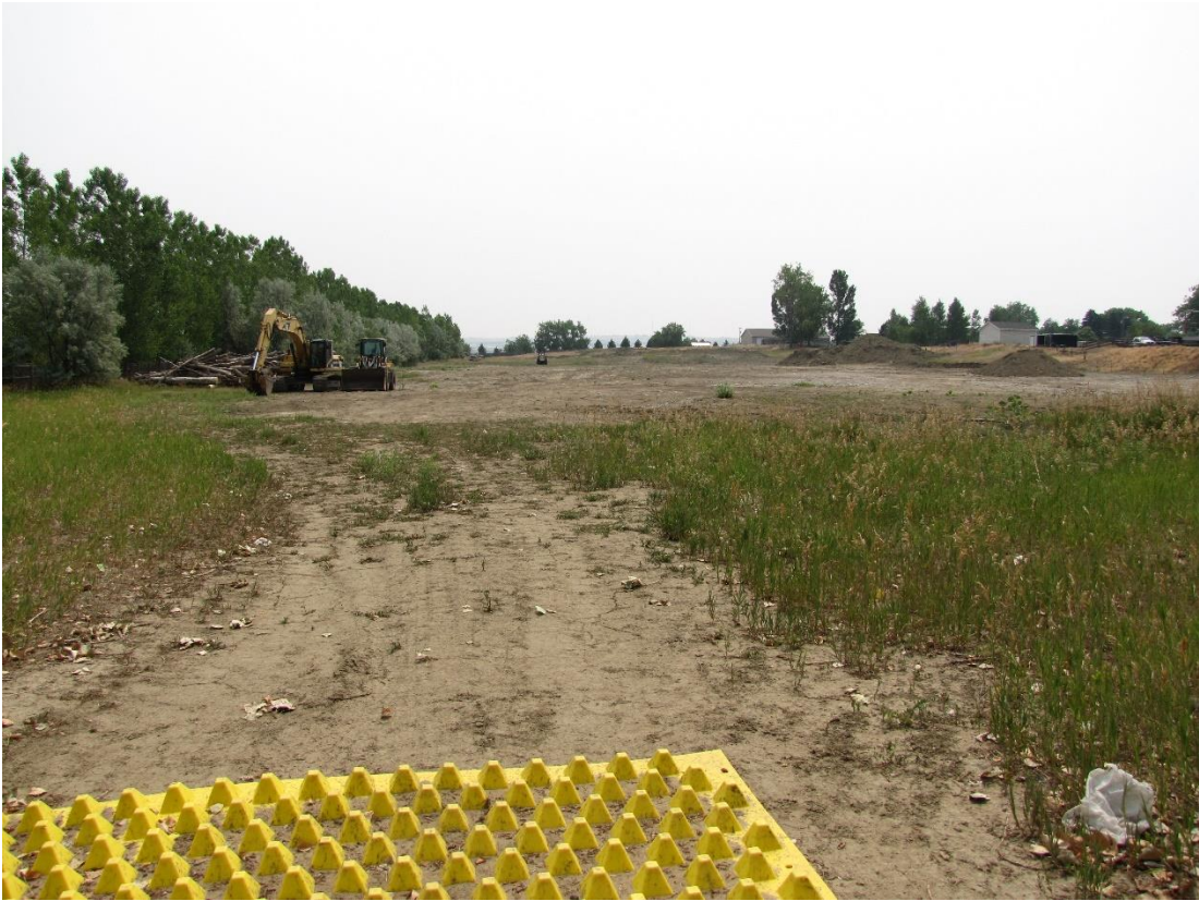
View south across subject property
