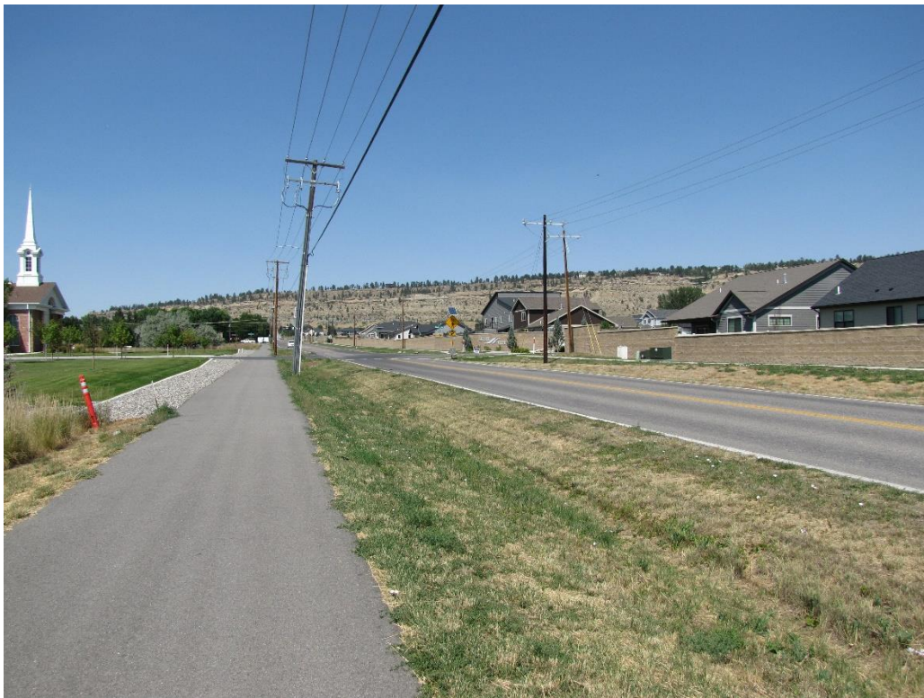
View north on 54 th St W
