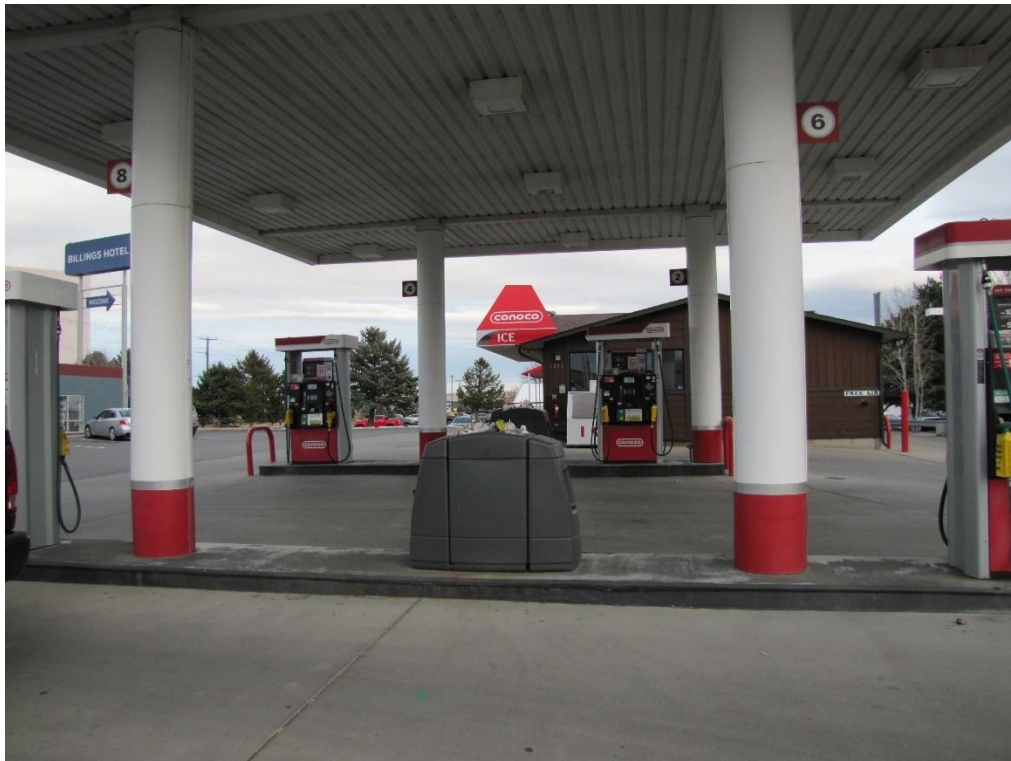
View east under fuel canopy to building to be renovated
