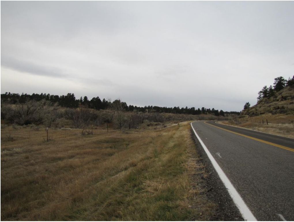
View west an Alkali Creek Rd
