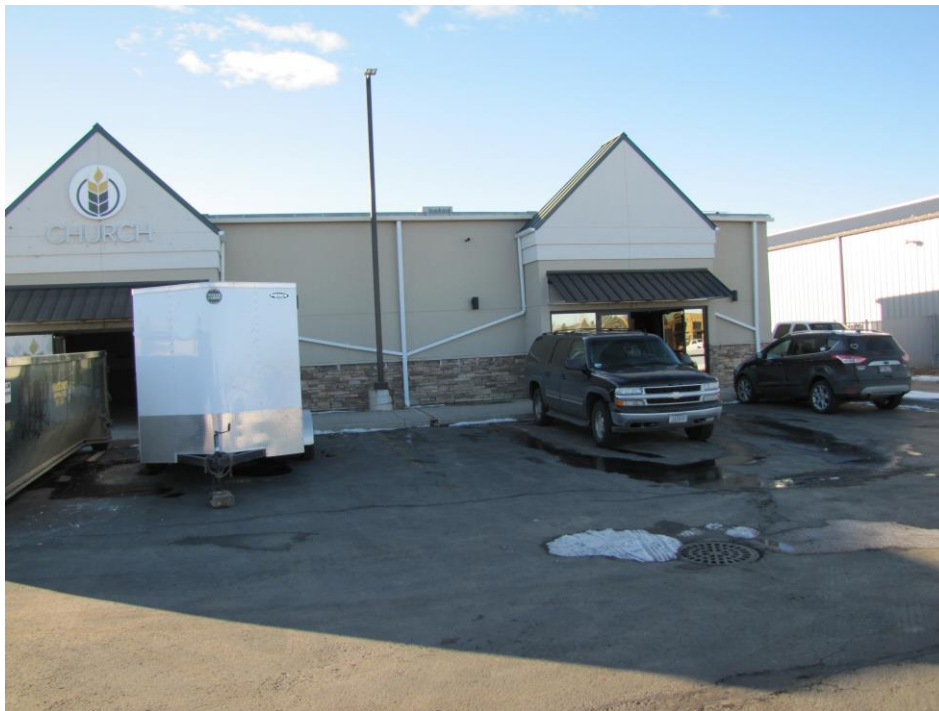
Looking Northwest- existing entrance
