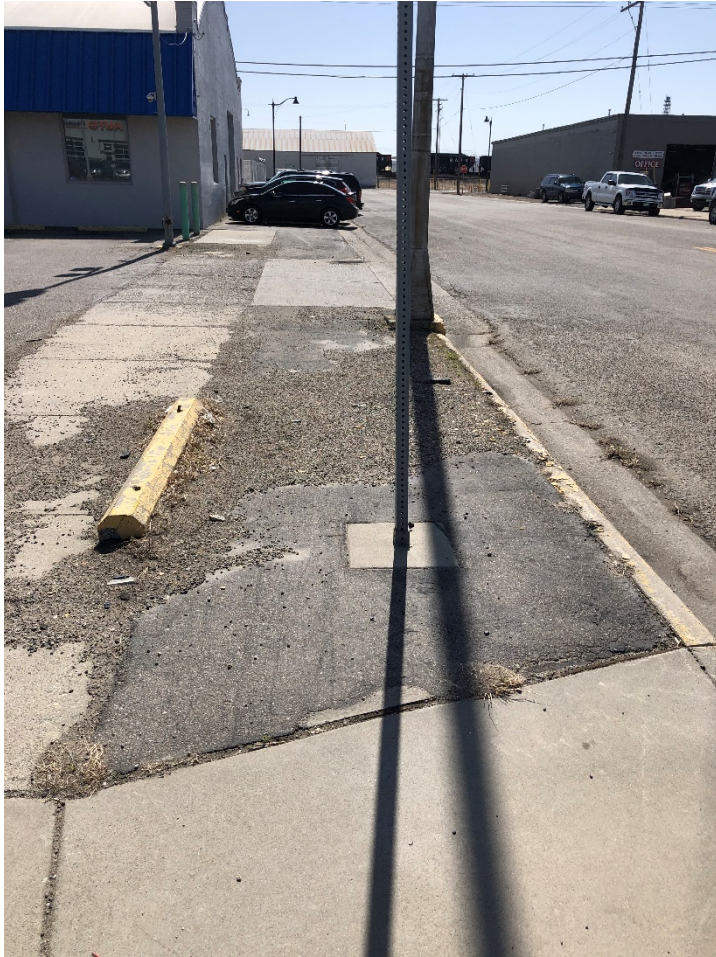
View along North 16 th Street property frontage with obstructions and unimproved boulevard area and sidewalk.
