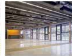
Overhead doors or sliding doors
