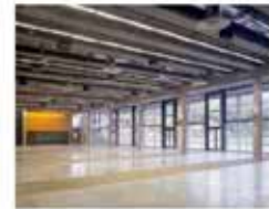
Overhead doors or sliding doors
