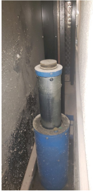
Oil buffers are code compliant
