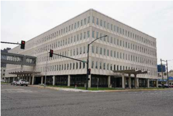
Photo #1 Overall view of the Stillwater Building looking southwest.
