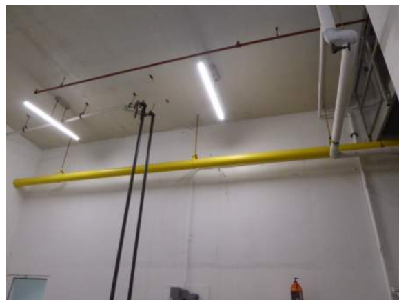
P16: sub basement wall cracks have been sealed
