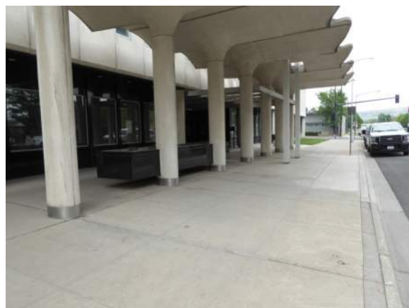
P4: east entrance canopy
