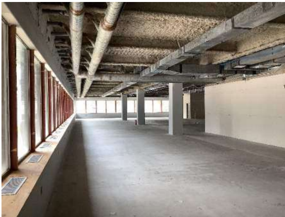
Photo #9 Overall view of the first floor at the time of our assessment.
