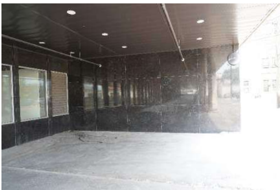
Photo #23 View showing the granite cladding at the top of the vehicular ramp.
