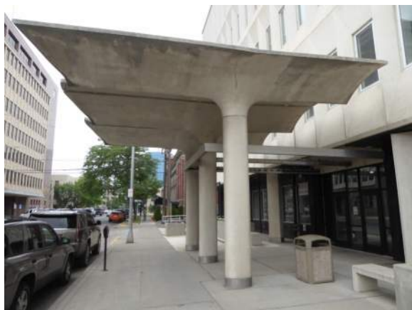
P1: south entrance canopy
