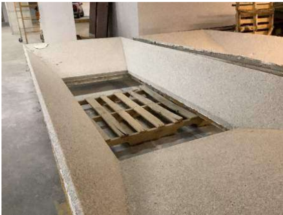
Photo #21 Wall panels removed from the façade and stored in the basement.
