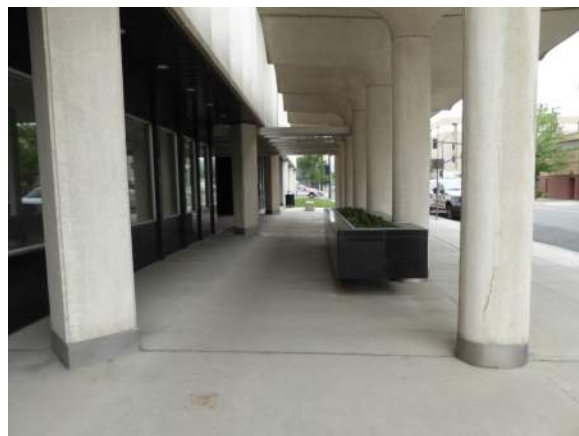
P2: east entrance canopy
