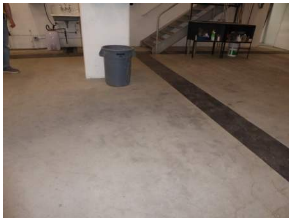
P13: sub basement
