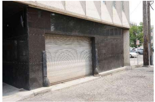
Photo #4 West elevation overhead door.
