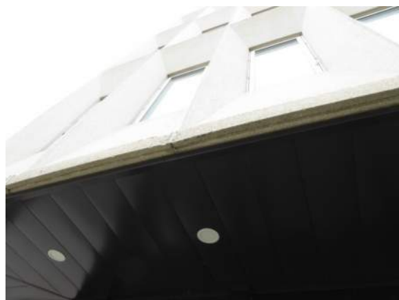
P6: weathered façade
