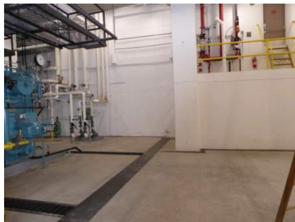
P18: sub basement
