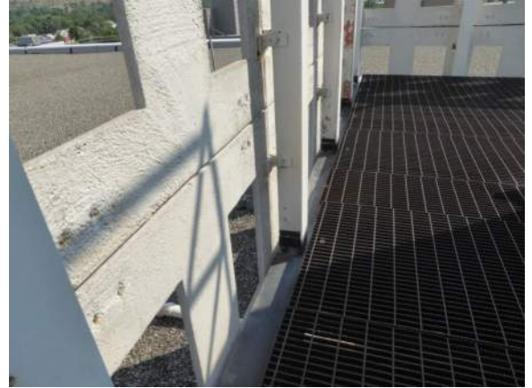
P40: Roof top mech equipment enclosure; precast concrete panels and steel frame
