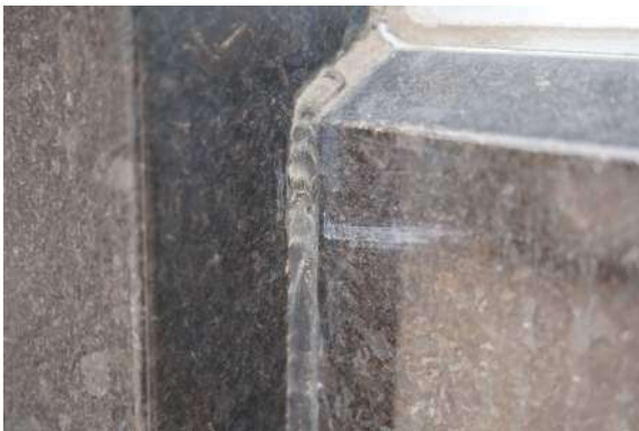
Photo #57 Sealant at the granite panels was typically not tooled but otherwise in serviceable condition.
