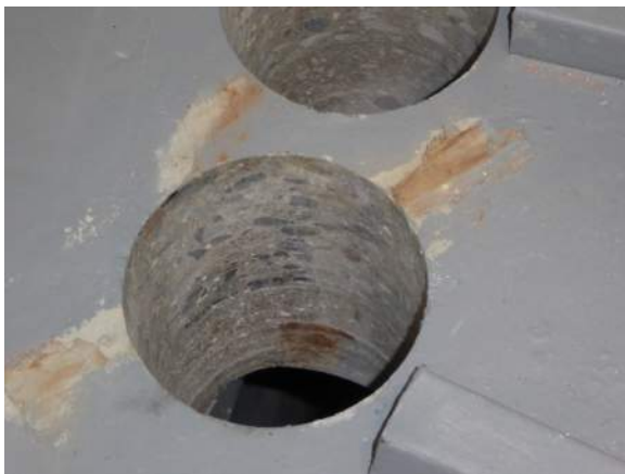
P11: slab on metal deck core holes
