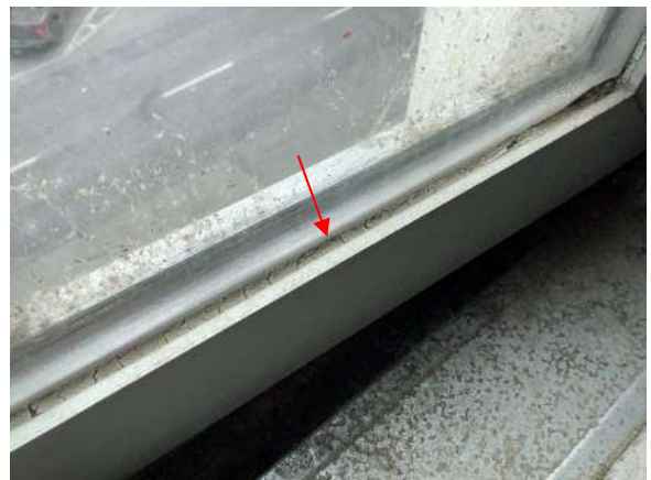
Photo #40 Condition of the exterior compound glazing at the open sash indicated by the red arrow.
