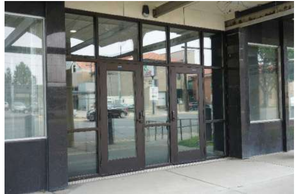
Photo #44 North elevation entry storefront. The south elevation entry storefront is similar.
