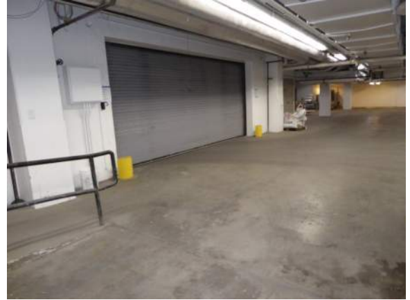
P8: basement garage
