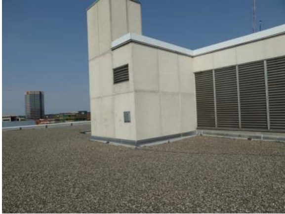
P39: Exterior façade at the roof penthouse
