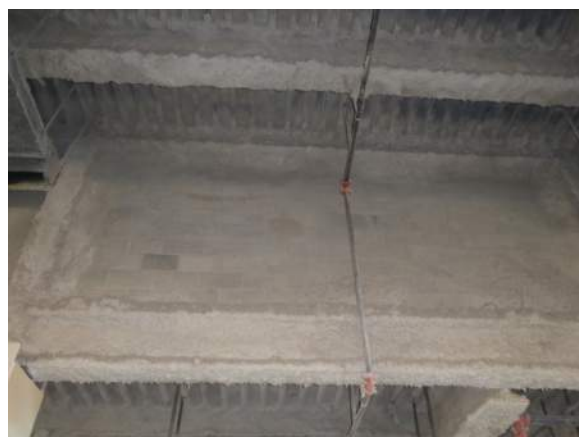
P38: Courtroom clerestory masonry infill with tight cracks likely from normal shrinkage
