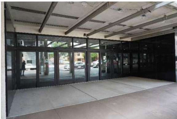
Photo #45 East elevation entry storefront.
