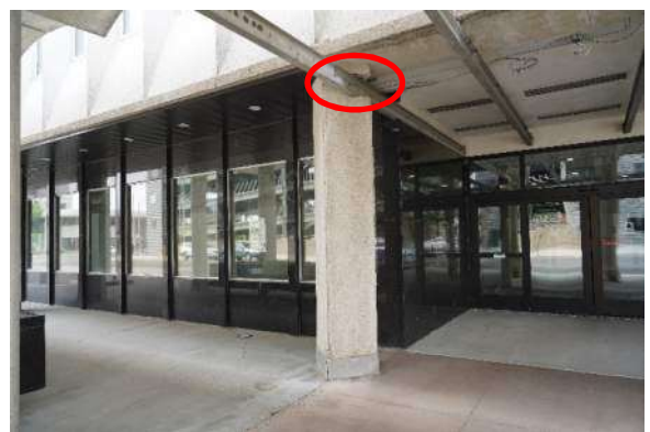
Photo #18 Column cover at the east entrance. Note the cover was modified to accommodate a beam indicated by red oval.
