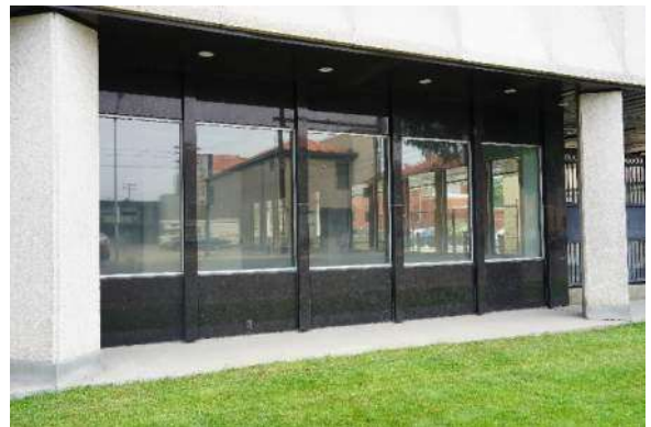
Photo #22 Typical view of the granite cladding installed at the first floor.
