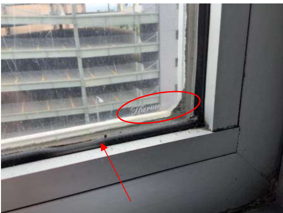
Photo #49 Original IG units have “Thermopane” etched in the lower right corner (red oval) and interior glazing gaskets (red arrow).
