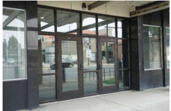
Photo #44 North elevation entry storefront. The south elevation entry storefront is similar.
