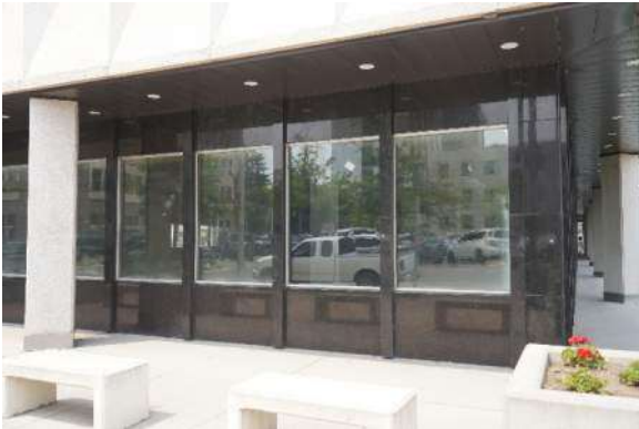
Photo #7 Polished black granite cladding at the first floor.
