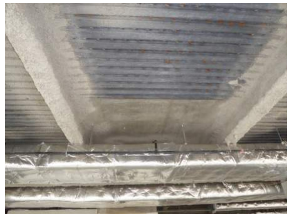
P12: typical slab on metal deck
