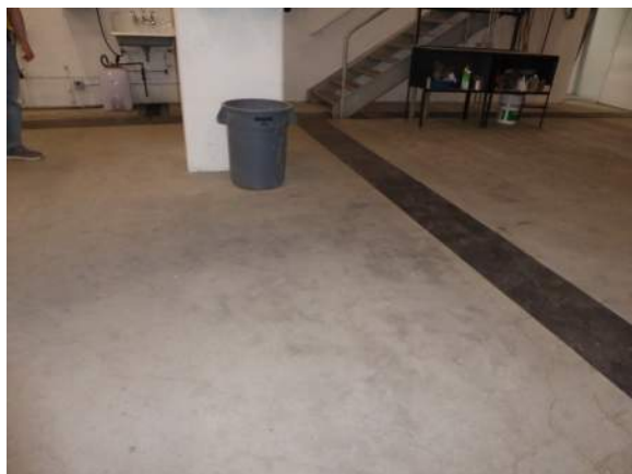
P13: sub basement
