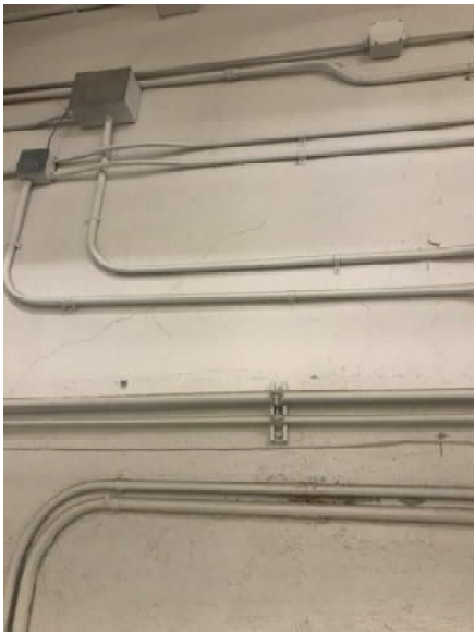
P28: concrete crack
