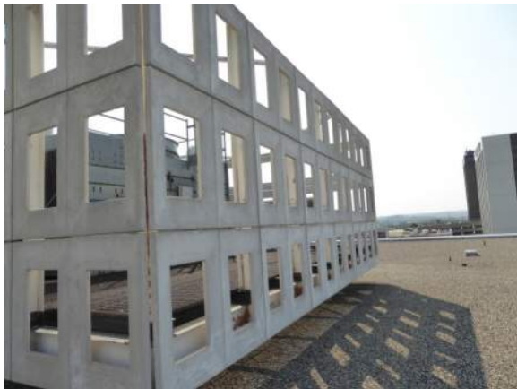
P41: Roof top mech equipment enclosure; precast concrete panels and steel frame
