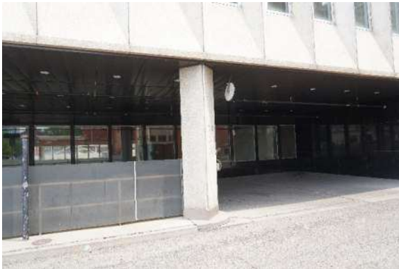
Photo #3 West elevation entry to the vehicular ramp to the basement garage.
