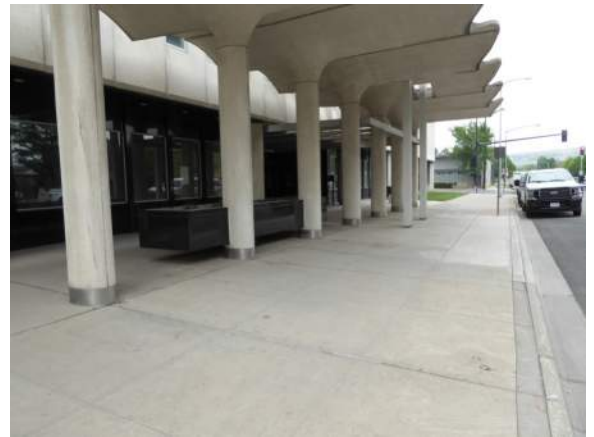
P4: east entrance canopy
