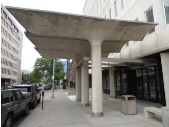
P1: south entrance canopy
