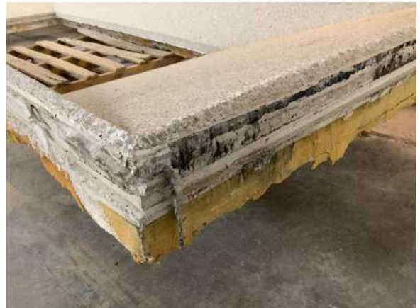
Photo #20 Wall panels removed from the façade and stored in the basement.
