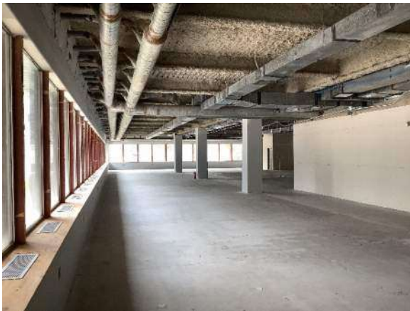
Photo #9 Overall view of the first floor at the time of our assessment.
