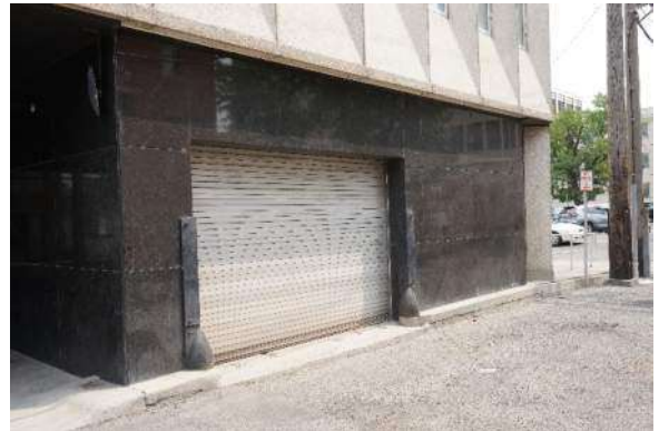
Photo #4 West elevation overhead door.
