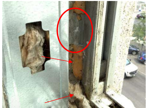
Photo #34 Batt & SPF insulation indicated by red arrows. Window anchor indicated by red oval.
