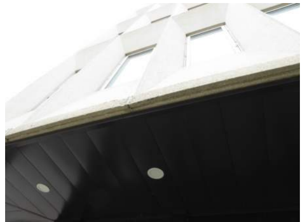
P6: weathered façade
