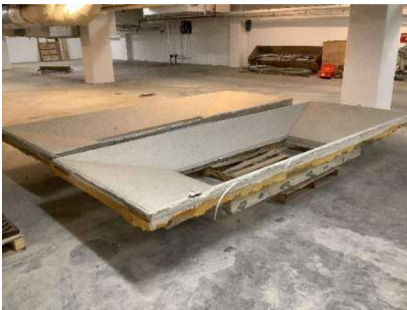
Photo #5 Precast panels removed as part of the pedestrian bridge construction.
