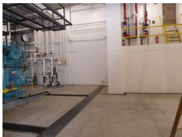
P18: sub basement
