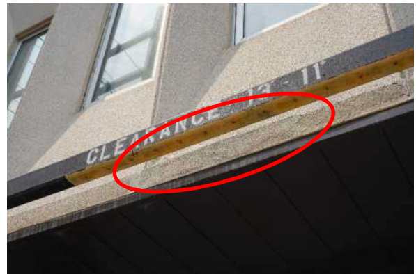
Photo #16 Area of concrete repair at the south elevation overhead door indicated by the red oval.
