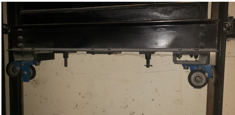
Counterweight rollers and rails are in good shape.
