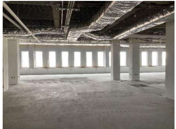
Photo #8 Overall view of the fifth floor at the time of our assessment.
