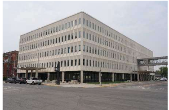
Photo #2 Overall view of the Stillwater Building looking northwest.
