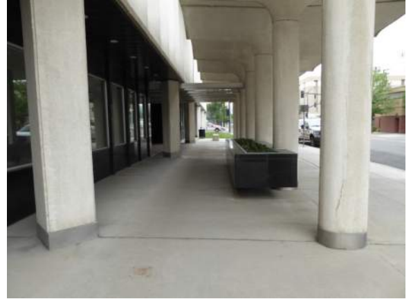
P2: east entrance canopy
