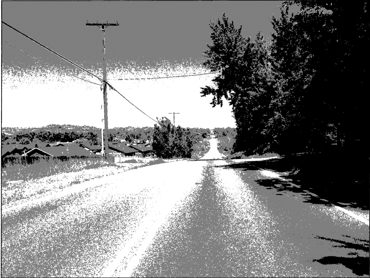
Attachment A Bitterroot Drive facing northerly
