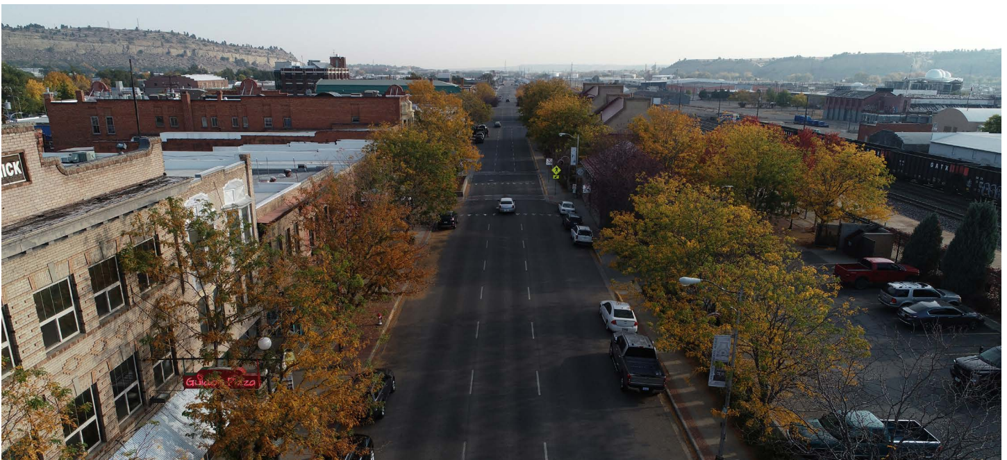
Montana Avenue currently has three one-way lanes with parallel parking on either side.
