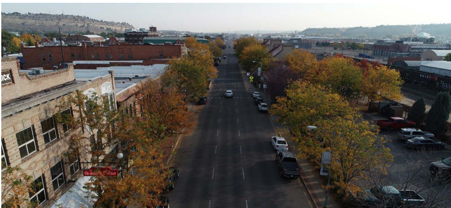
Montana Avenue currently has three one-way lanes with parallel parking on either side.
