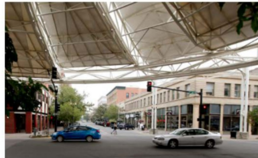
Traffic moves east on Second Avenue North under Skypoint in downtown Billings. The street is one of the one-way streets in downtown that is being studied for possible two-way conversion, as well as a seasonal closure of the 100 block of North Broadway, pictured.
