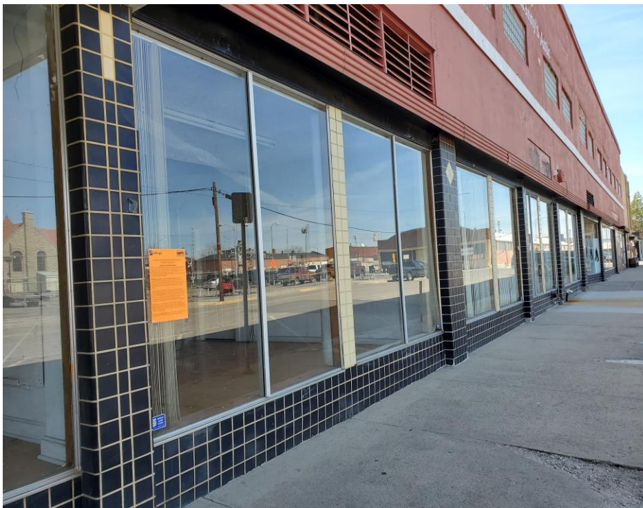
View west along storefront
