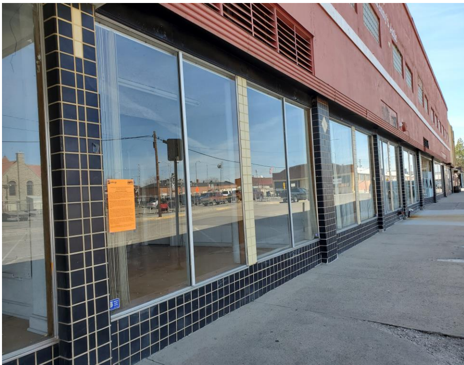
View west along storefront
