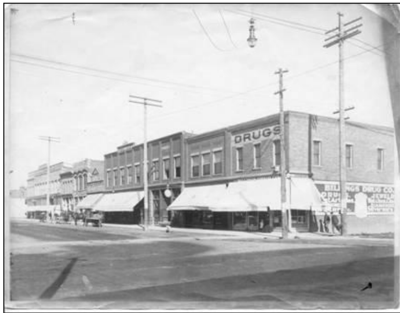
Yegen Block, c 1900, looking east from South 29 th Street
