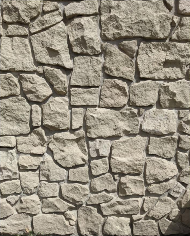
Sandstone Wall/ Column Material
