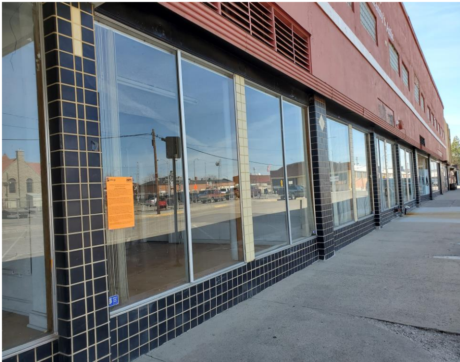
View west along storefront
