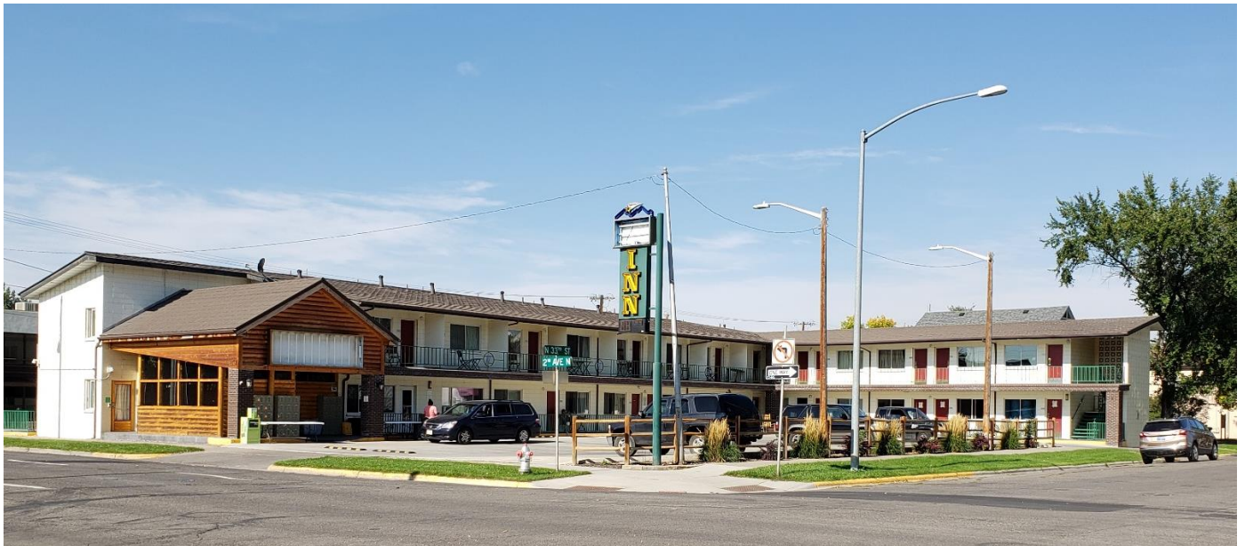
Subject of photo: 3311 2 nd Avenue N, Billings, MT 59101 Photo is taken looking: Northwest from the intersection of 2nd Avenue N & N 33 rd Street
