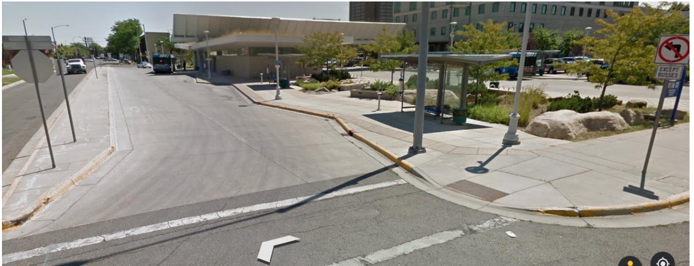
Subject of photo: 220 North 25 th Street, Billings, MT 59101 Photo is taken looking: Southwest from 2 nd Ave N & N 25 th St intersection
