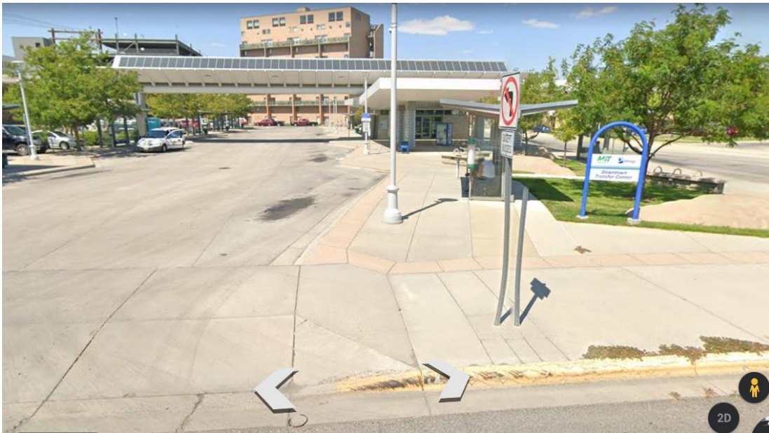
Subject of photo: 220 North 25th Street, Billings, MT 59101 Photo is taken looking: North from 2 nd Ave N
