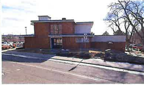
Structure to be Demolished
