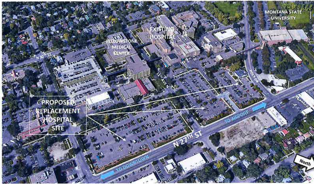
Existing Condition of Overall Project Area
