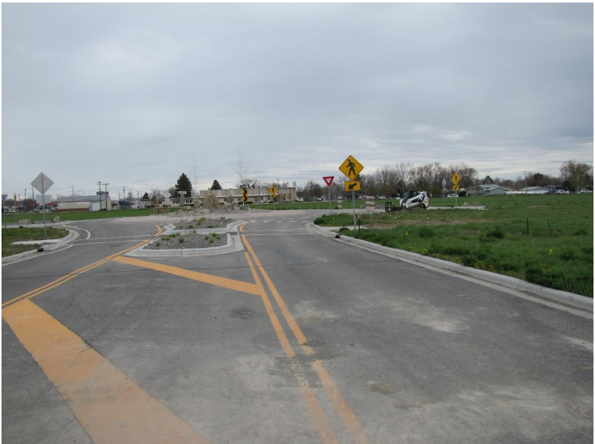
Looking East from the North side of the parcel
