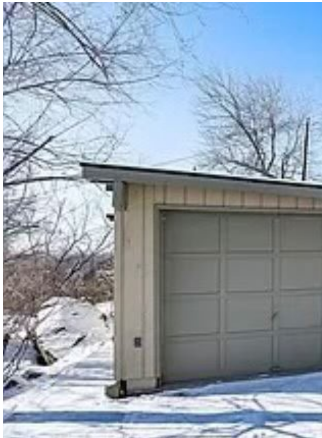
Applicant Photo of existing garage
