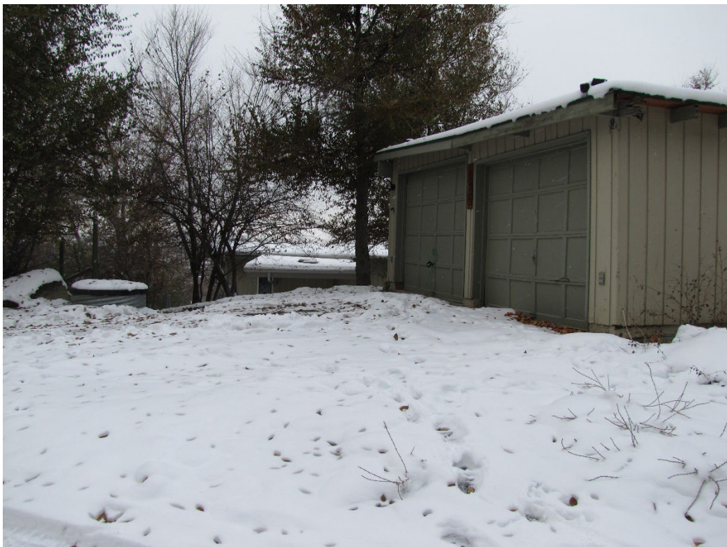
Existing garage – dwelling below and to the left
