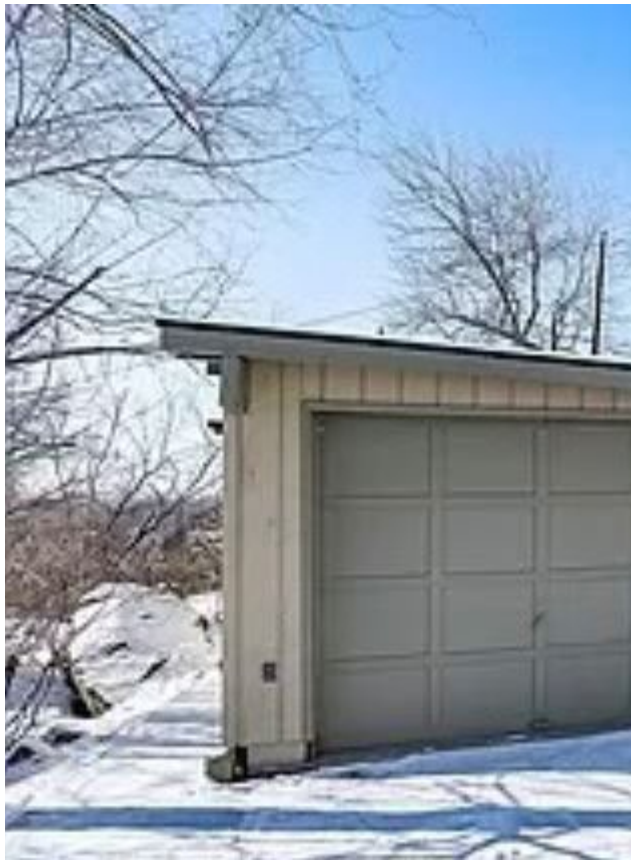
Applicant Photo of existing garage
