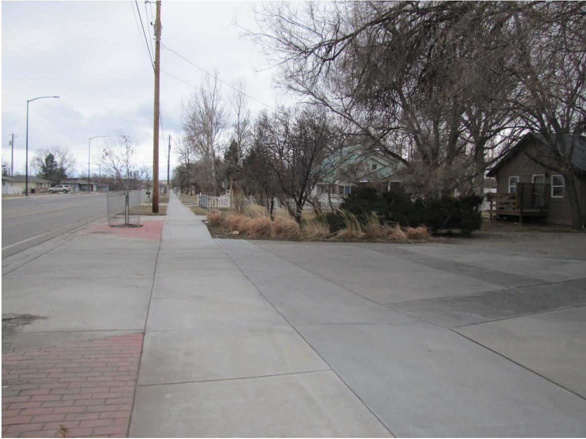
Looking South on Bench
