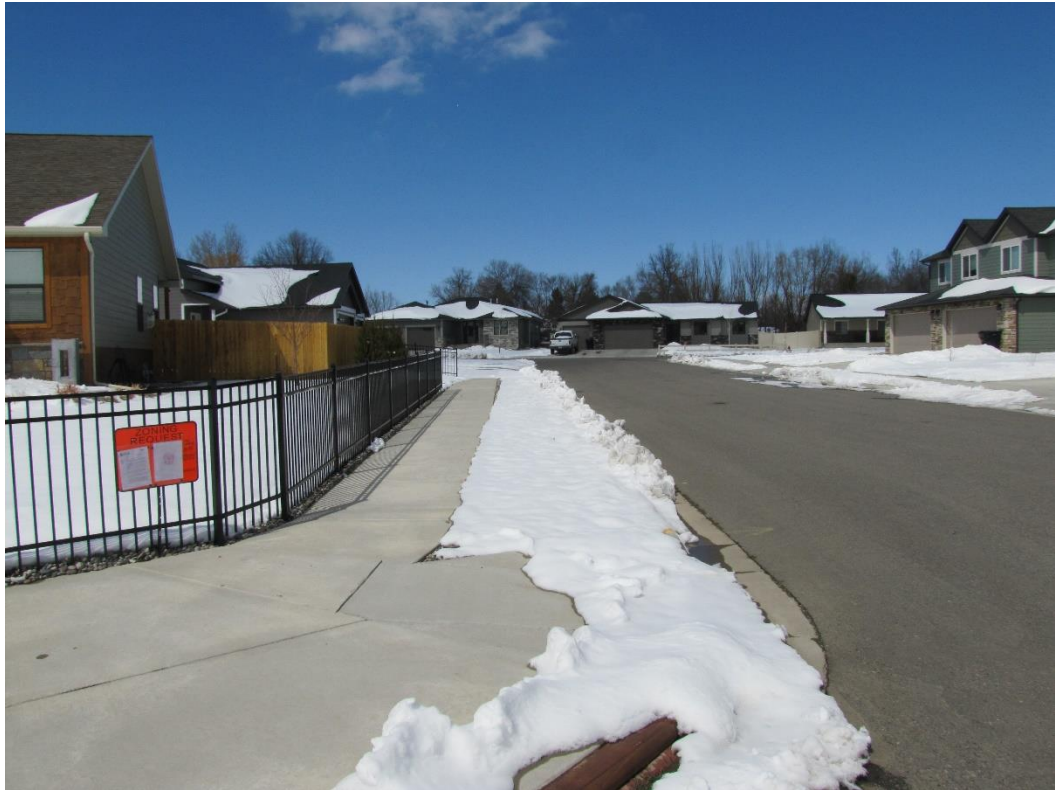
Looking North on Columbine
