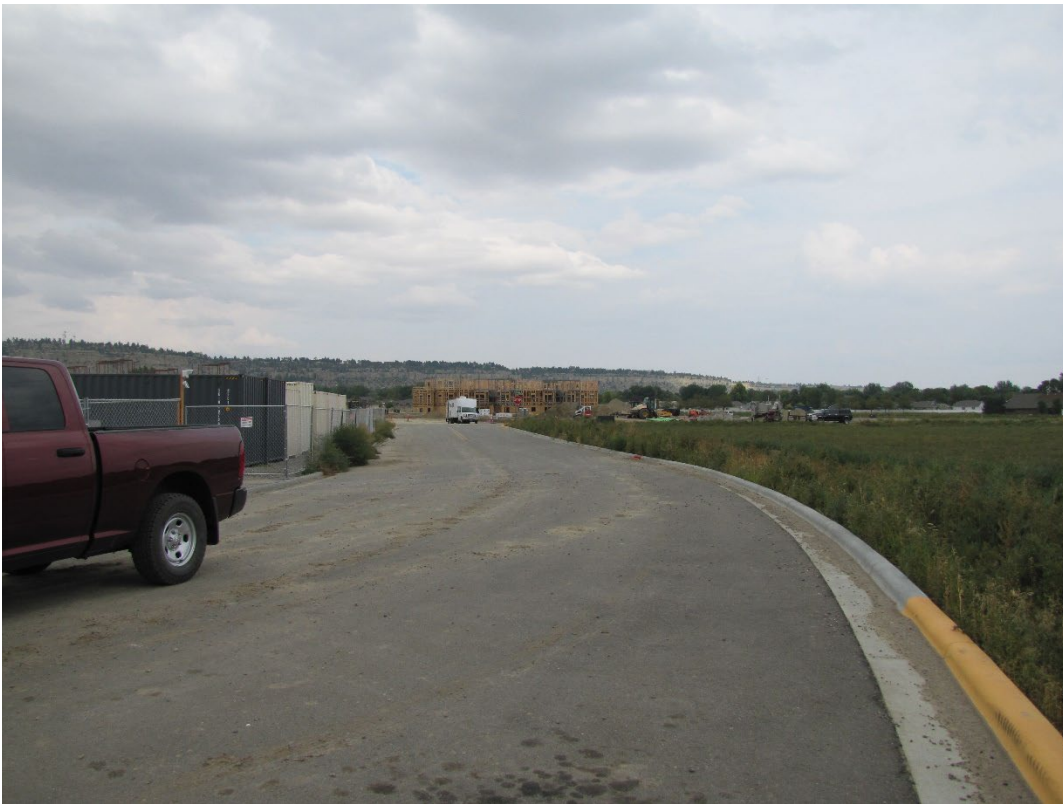
View north to apartments under construction in Zimmerman Home Place
