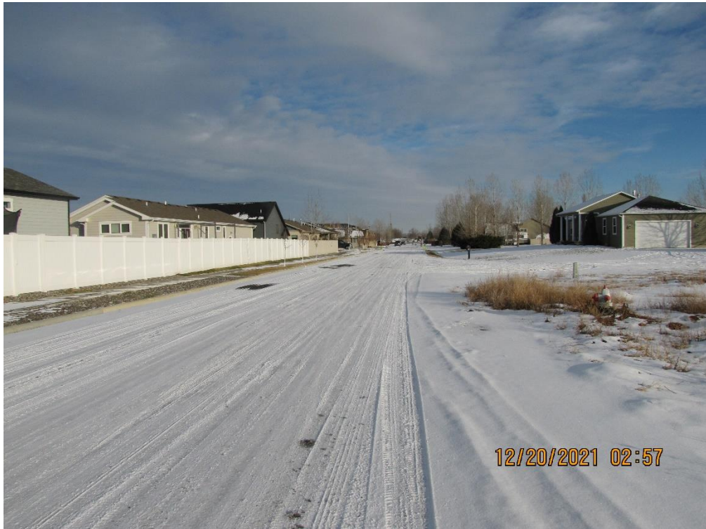
View east on Bell Ave at NW corner of subject property
